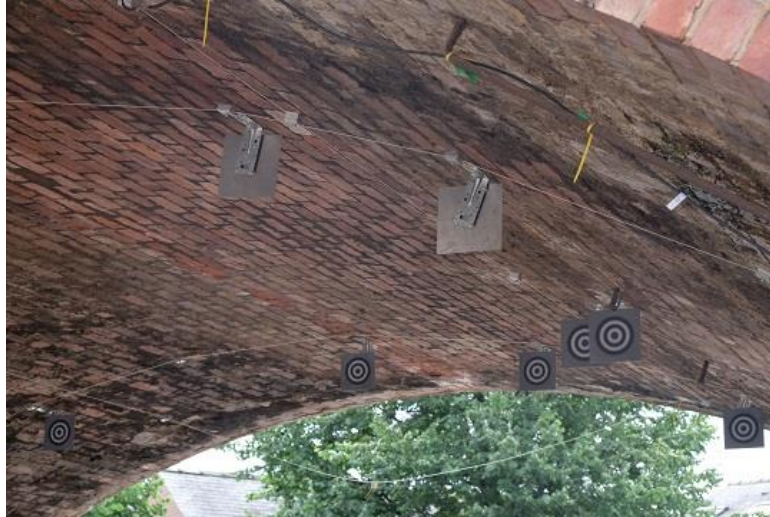
Figure 5: Examples of the videogrammetry targets used at Marsh Lane viaduct.
