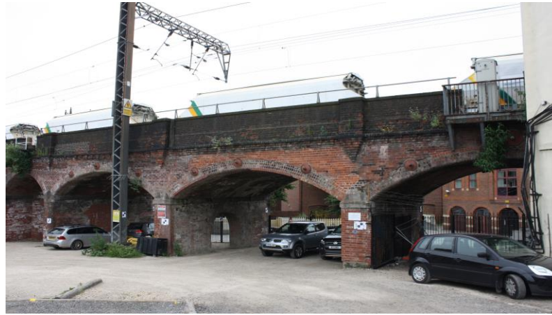
Figure 1: The Marsh Lane viaduct.
