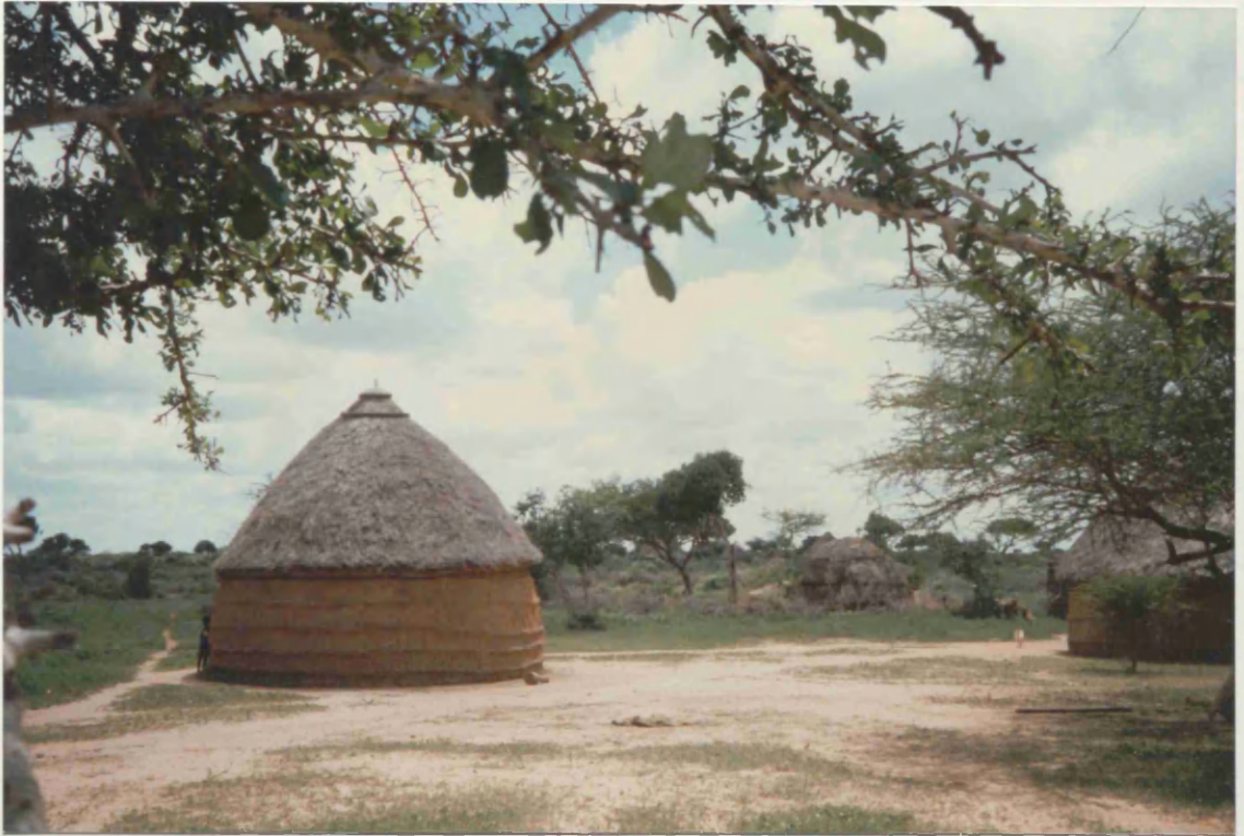
Plate 6.3 A permanent mundul (singular of mundullo) hut. It has a rounded base with the lower part covered by wattle and daub. The roof is conical in shape and thatched. This type is quite common amongst the agro-pastoral groups of Bay region.
