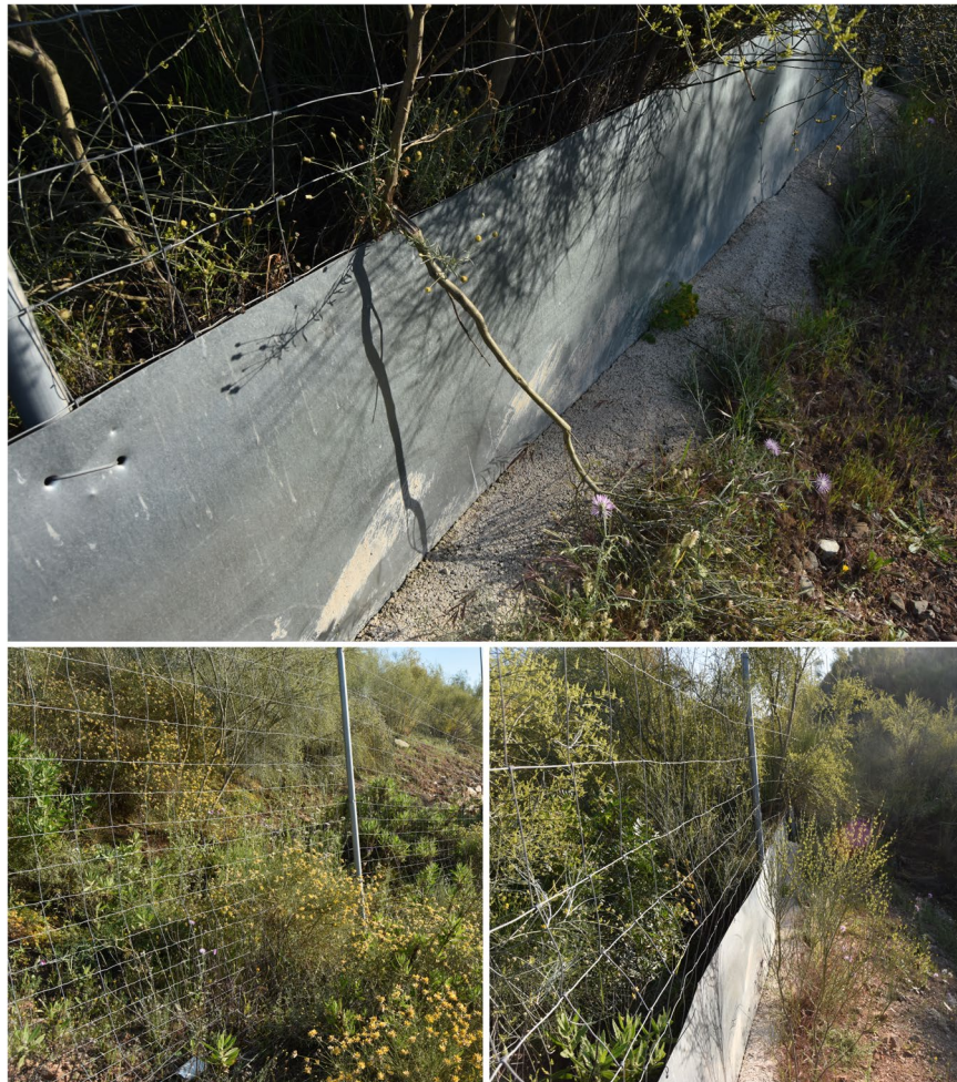
Figure 2. Top image: reptile fence. Left image: chain link fence without metal sheet. Right image: reptile fence with vegetation around it.
