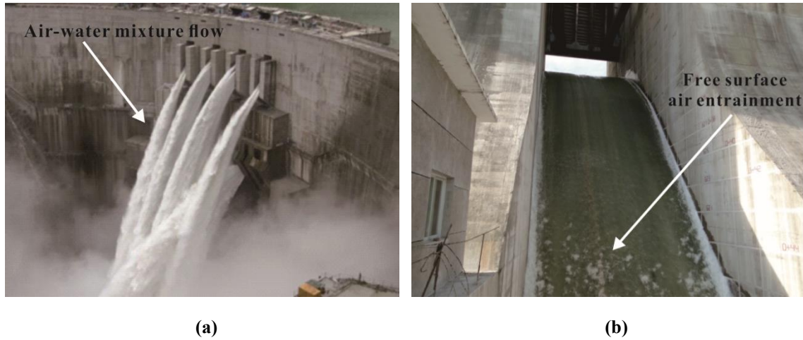
Fig. 1. Air–water flows in hydraulic engineering: (a) Jinping-I dam; (b) Wudu spillway (photos taken by Professor Jun Deng).
