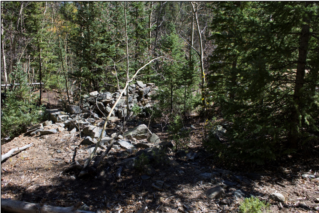
Figure C- 11. Hall Valley, Feature 9 collapsed stone wall/foundation, view southwest.
