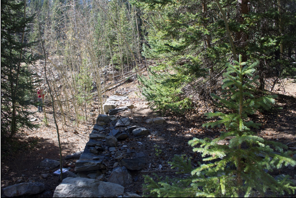
Figure C- 14. Hall Valley, Feature 11 view of platform atop smelter foundation wall view west.
