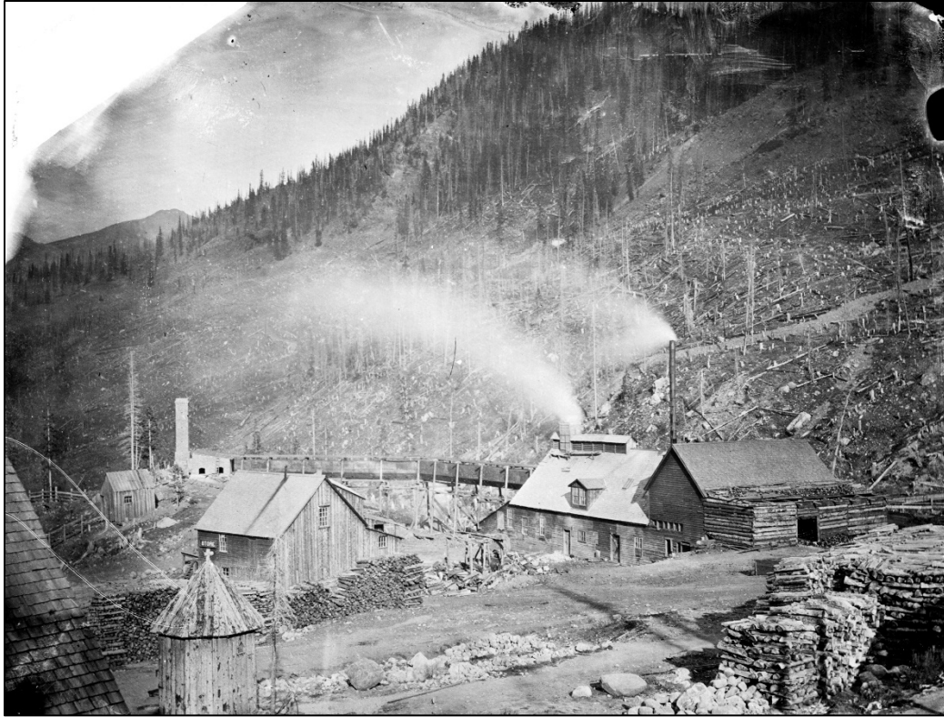
Figure 3-9. Smelter at Sts. John ca. 1870-1880 showing furnace in left background, roaster in right mid-ground, and piles of cordwood at lower right. Colorado Historical Society X-13495
