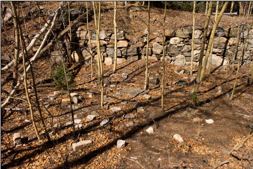
Figure C- 15. Hall Valley, Feature 11 view of interior smelter wall with scattered common and fire brick in foreground.
