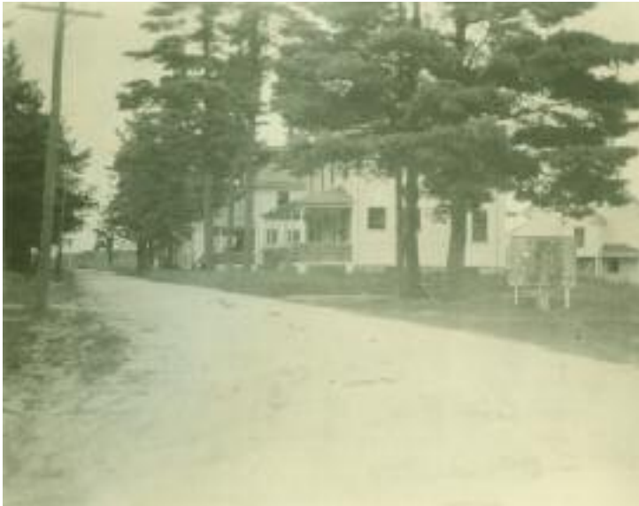
Box Shop (above) and village street (below) at E.I. DuPont's Smith's Mills property in Standish, 1923. In its heyday during WWI, Smith's Mills employed hundreds of men and produced 40,000 feet of lumber daily to support the overseas war effort. The Portland Water District, calling Smith's Mills "one of the worst dangers of pollution about the lake," purchased the property for $90,000 in 1923, and subsequently razed or relocated every building on the property, returning it to a forested state. Images courtesy of the Portland Water District.
