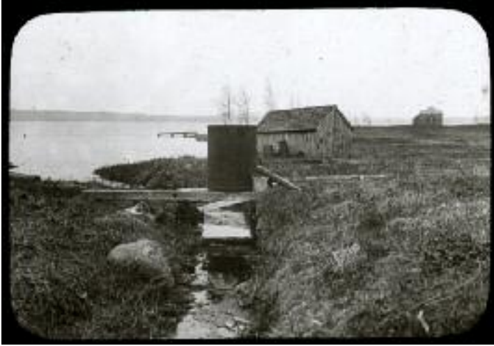
Temporary hypochlorite plant at Hinkley Brook in Standish, 1916. The plant was deployed to chemically treat water from the polluted tributary, before it entered the lake near the District's intake. Image courtesy of the Portland Water District.
