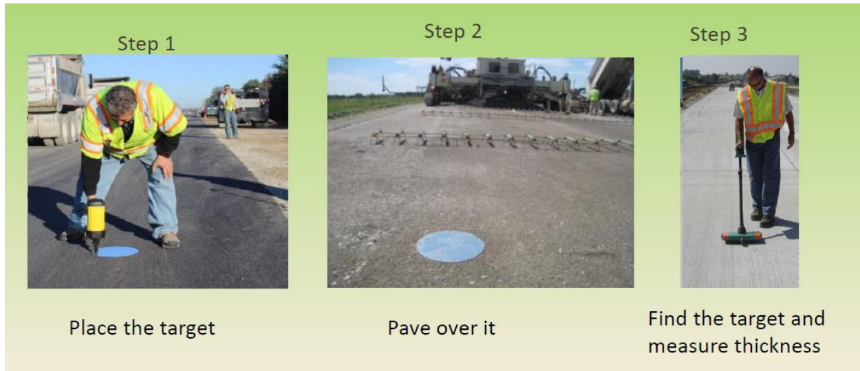
Figure 6 Steps for Using the T2 (Ref. TRB 2268)
