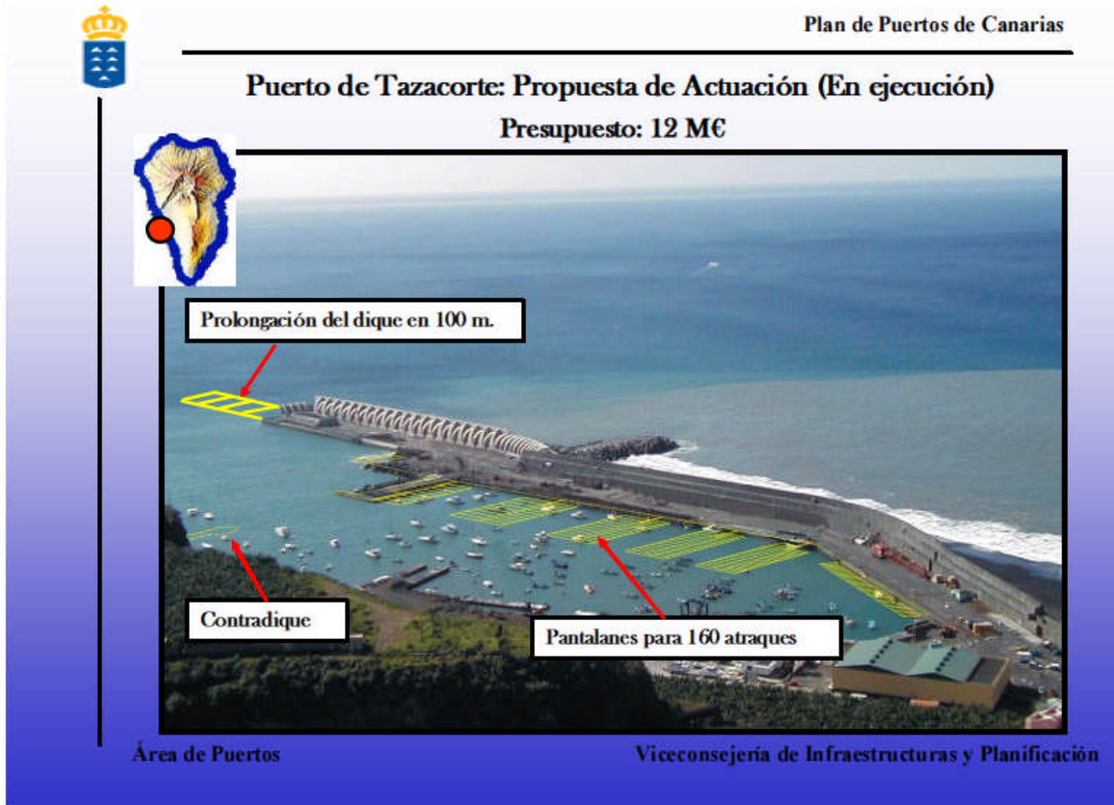
Figure 11 Port of Tazacorte – In between 2000 and 2006
