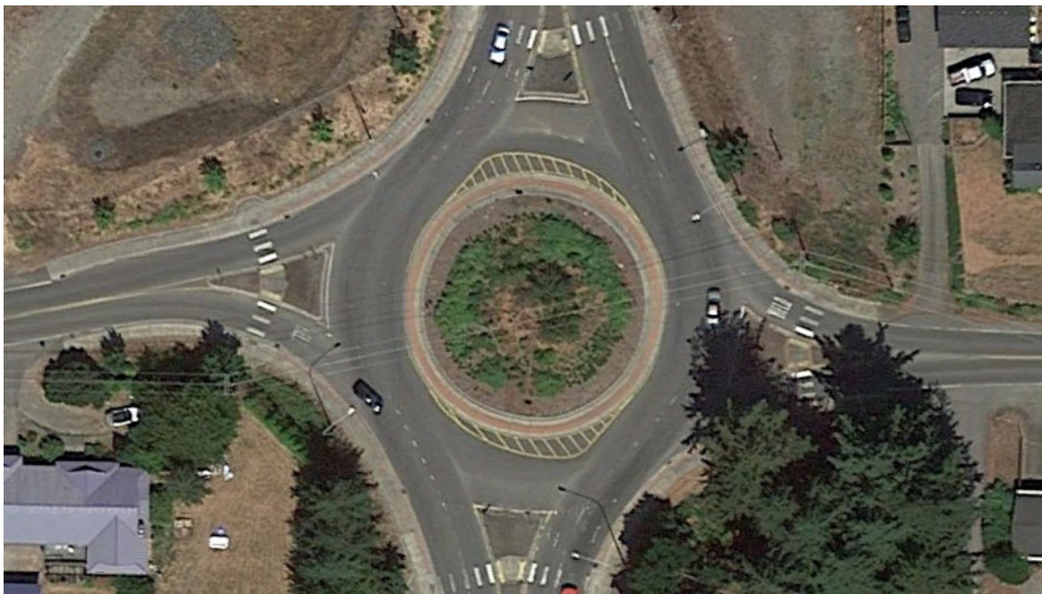
Figure 5.1 Roundabout junction of highways 539 & 544 southwest of Lynden, WA [22]
