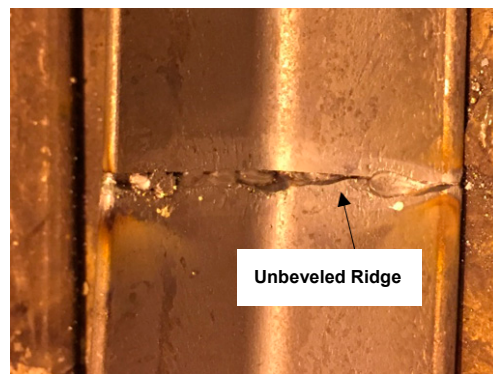
Figure 4. Manufacturing cracks in the welds by leaving out a part of the bevels.
