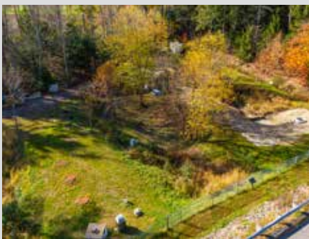
The University of New Hampshire Stormwater Center Field Site, adjacent the university’s West Edge Parking Lot. The site is designed to provide an apples to apples comparison of how stormwater treatment systems reduce pollution and manage the volume of runoff.
