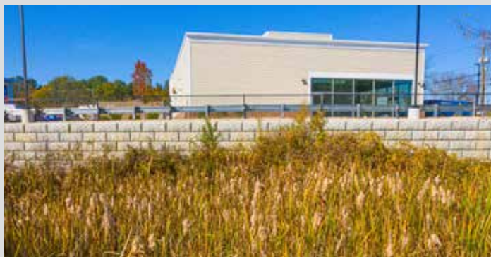
Filtration systems like this subsurface gravel wetland fit seamlessly into the landscape and improve water quality.
