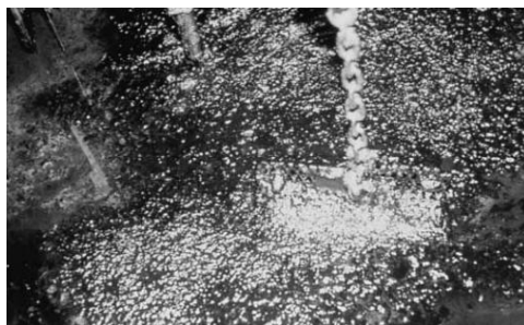
Fig. 1. Example of sludge build-up at the bottom of a fuel storage tank.
