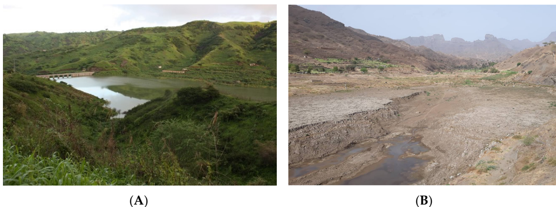
Figure 6. Poilão dam in São Lourenço dos Órgãos at the Santiago Island (A) Rainy season; (B) Dry season). Photos taken by the authors (MMR and APE).
