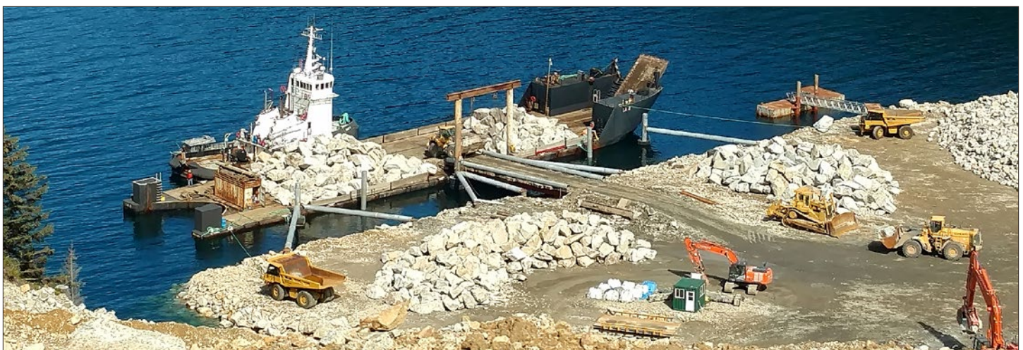
St. George Breakwater Storm Repair, Brice Inc.
