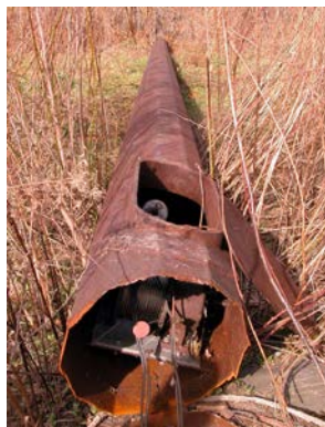
Figure 2.1: High-mast failure in Iowa
