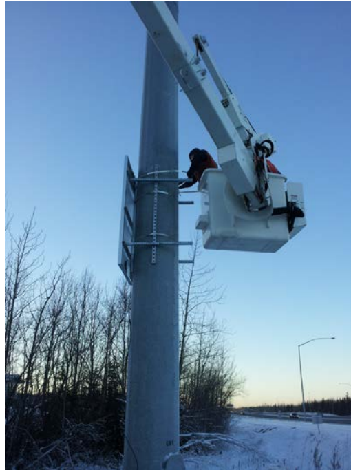
Figure 4.7: Solar Panel Installation at Weighstation
