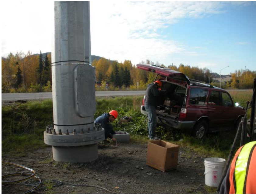
Figure 3.2: HMLP foundation connection at Peter's Creek
