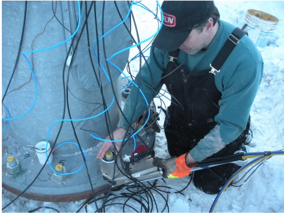
Figure 4.9: Rod Blohm (AKDOT&PF Bridge Crew) turning an Anchor Nut 20 Degrees
