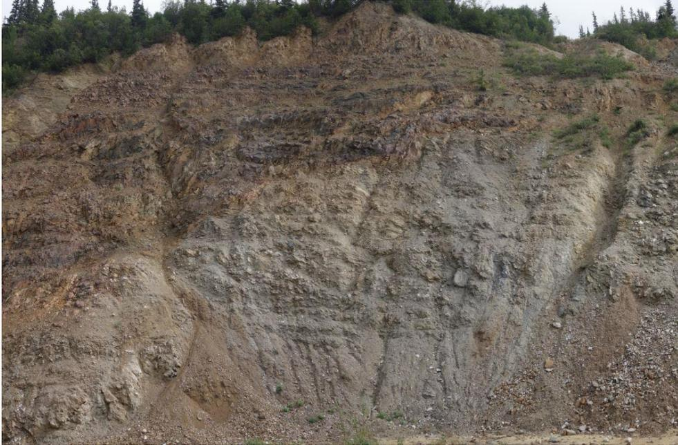
**Figure 4** Glitter Gulch rock slope with darker basalt and lighter schist
