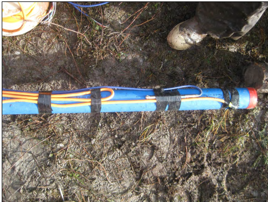
Figure B-6. Configuration of the piezometer and thermistor bead at the bottom and outside of the casing installed in TH12-9004. (Photograph by M. Darrow)
