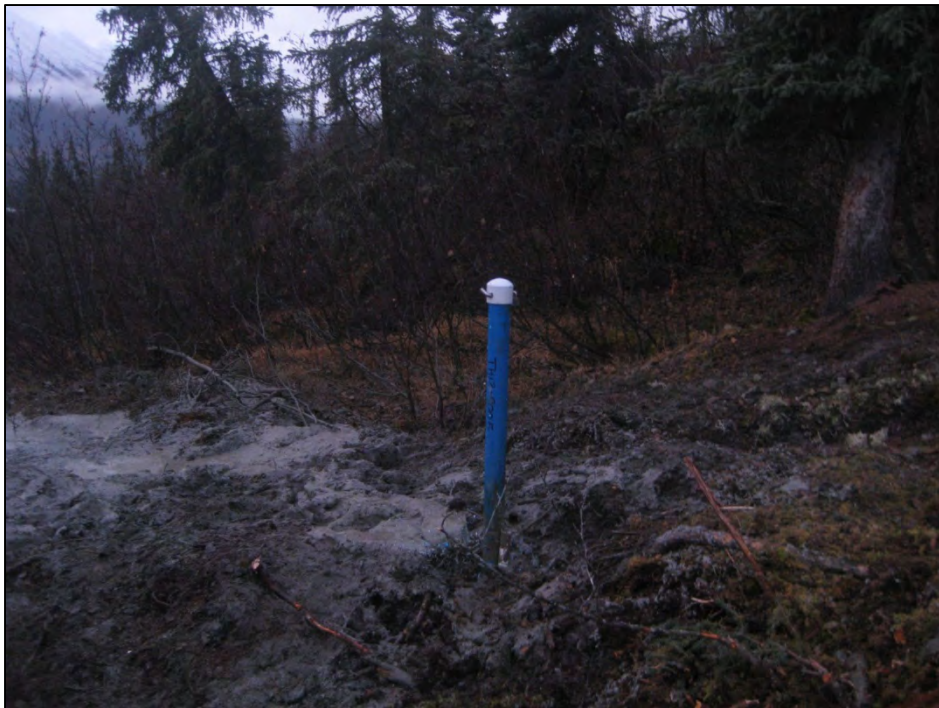
Figure B-10. Completed casing installation for TH12-9005. (Photograph by M. Darrow)
