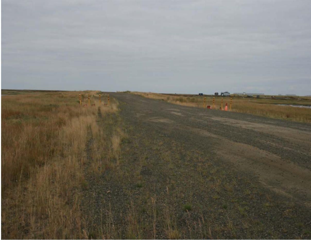
Figure 2: Elevated northern section of runway unused for airline traffic
