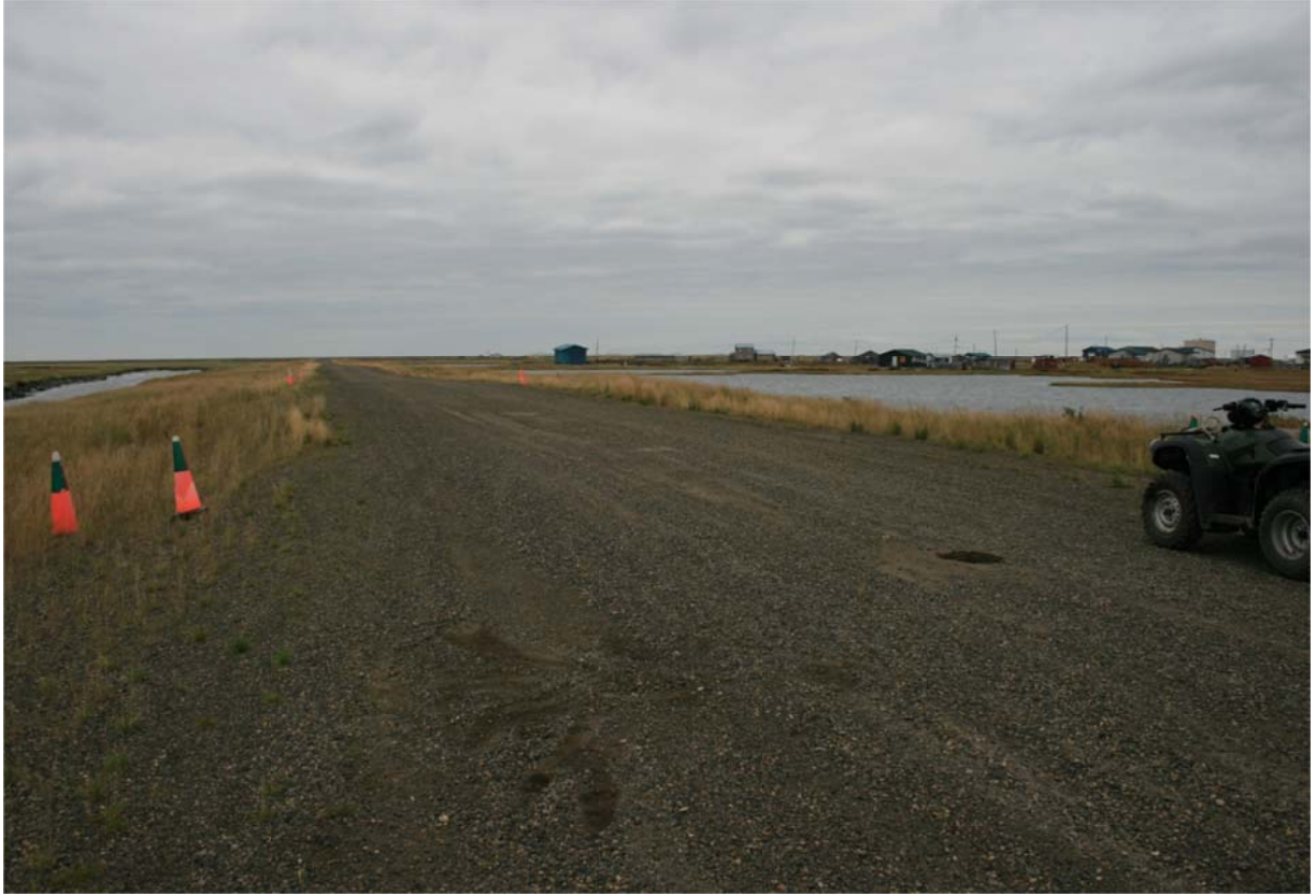
Figure 3: Area disturbed in front of picture is where eight inches gravel was found
