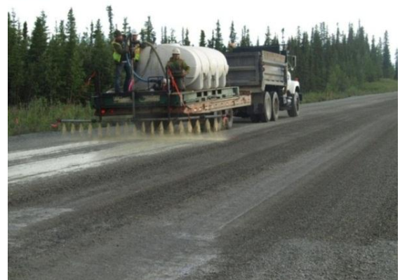
Figure 3 – Applying the palliatives with a 15' spray bar.
