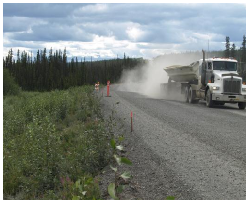
Figure 4 –Section 3A – 7/18/2011 –One day after application of Durasoil . (Note the difference in levels of dust generated by the two vehicles traveling at the same speed)
