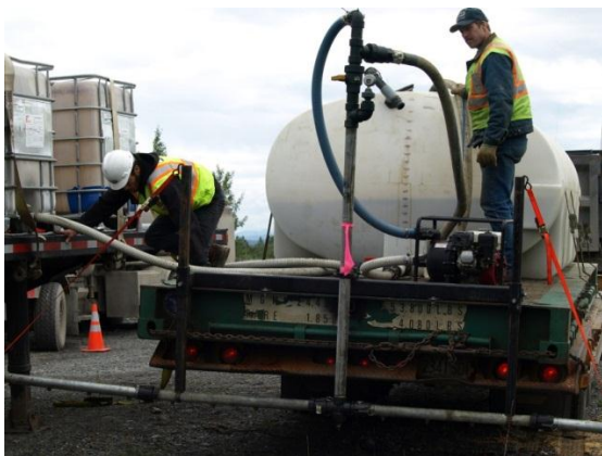
Figure 2 – Mixing palliative with water
