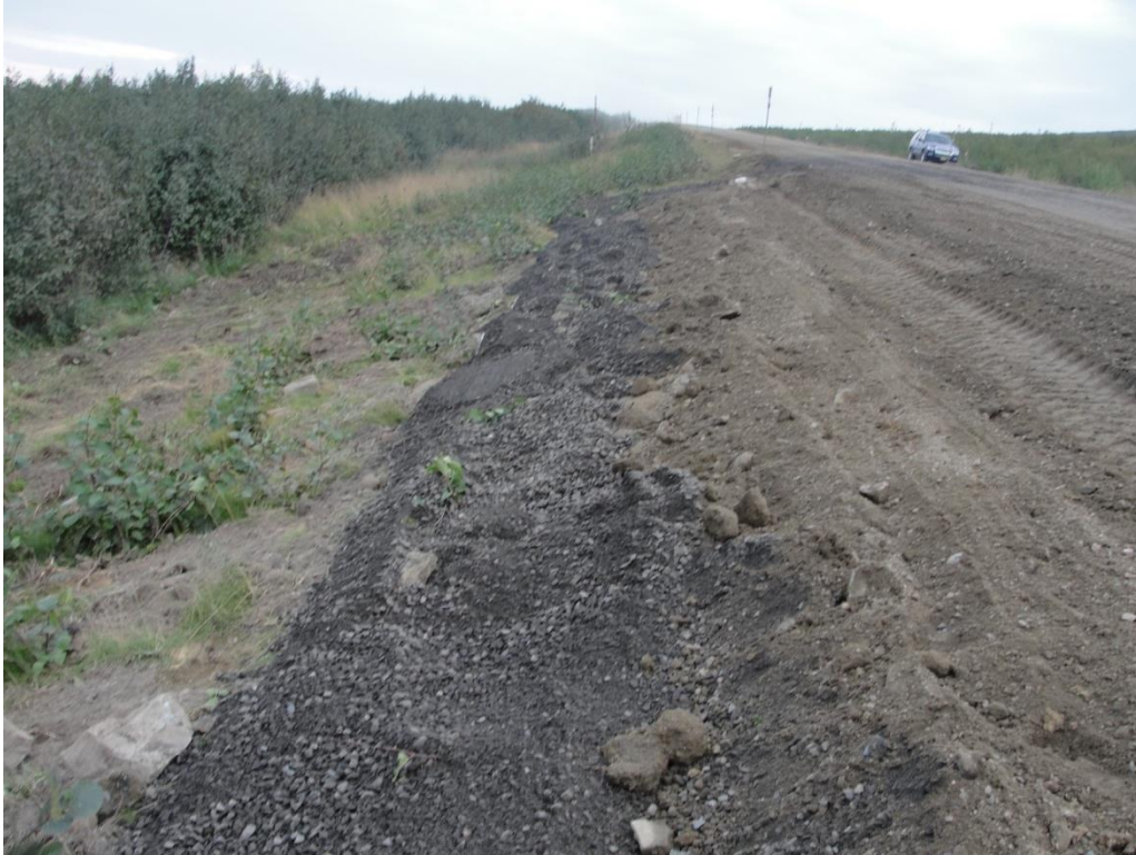
Figure 44. Test section after completion of construction
