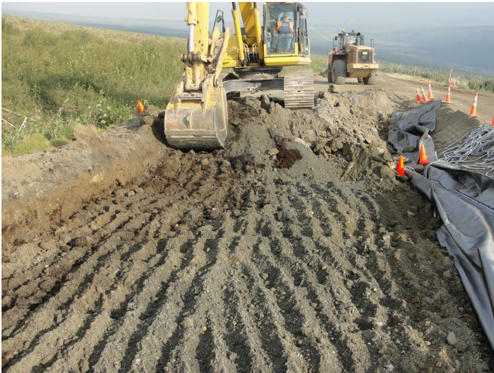
Figure 32. Excavation of the lane on the west side of the road
