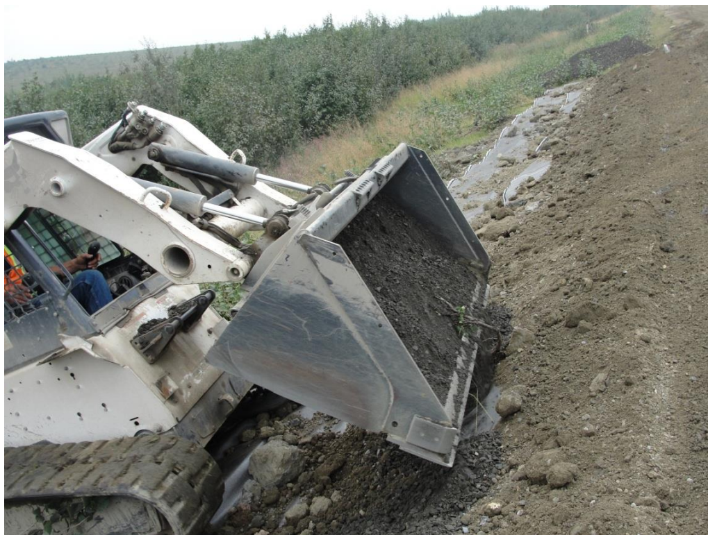
Figure 43. Covering the wicking fabric with crushed rocks
