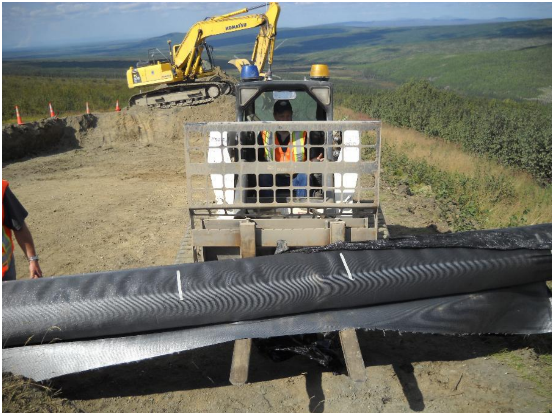
Figure 26. Wicking fabric was brought into the excavation area
