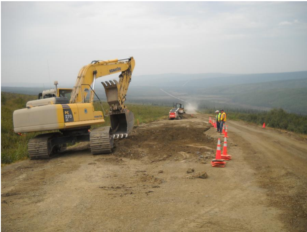
Figure 42. Backfilling the excavation area to its original elevation
