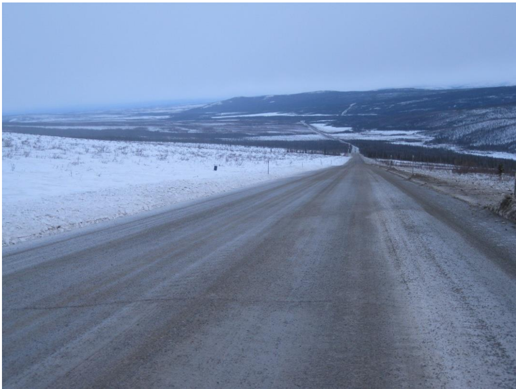
Figure 56. Site conditions on March 30, 2012
