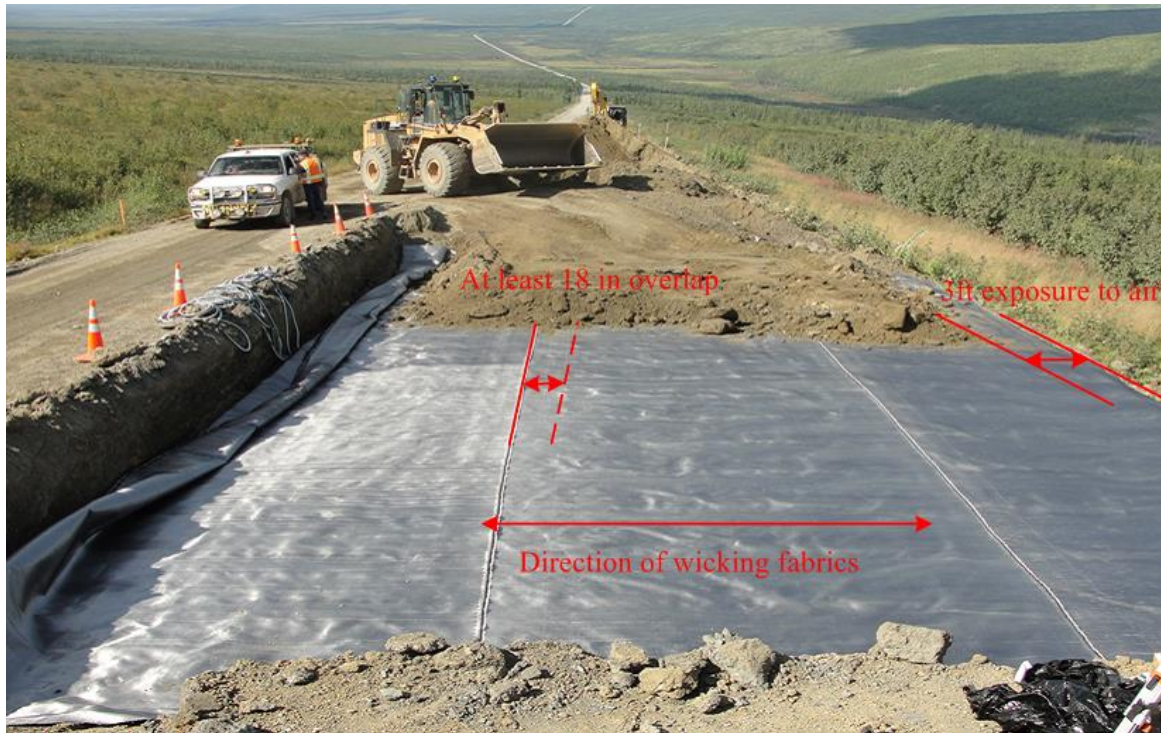
Figure 27. Wicking fabric installation after placement
