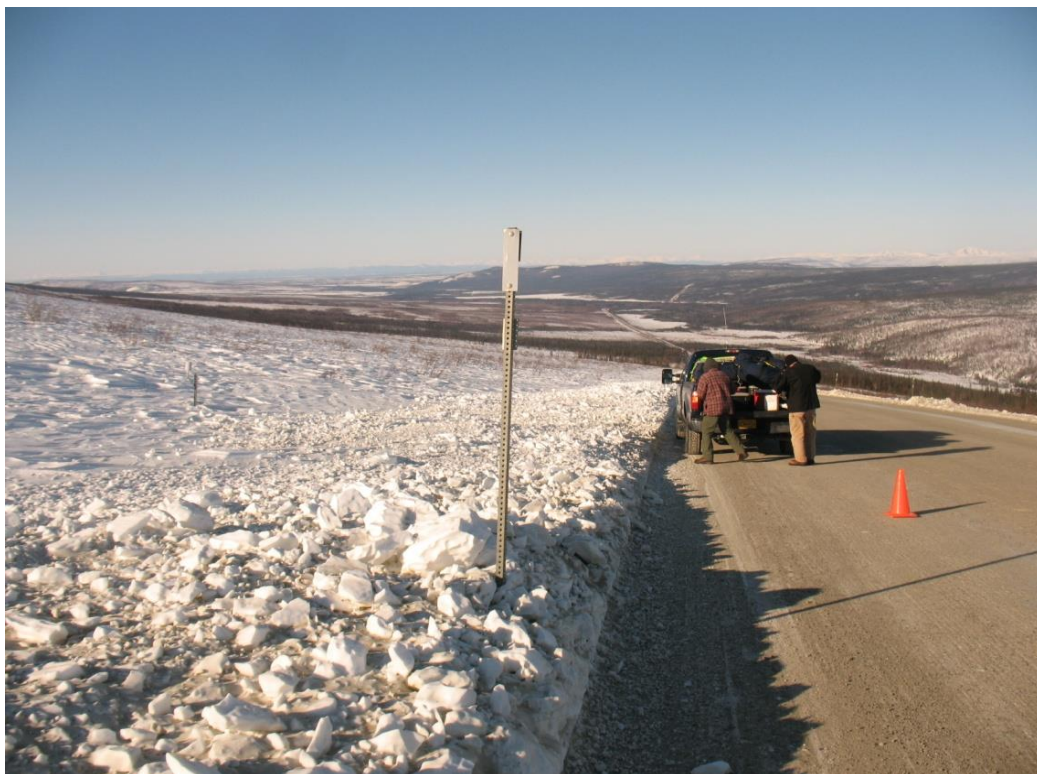
Figure 54. Site conditions on March 12, 2011, before installation of the solar panel
