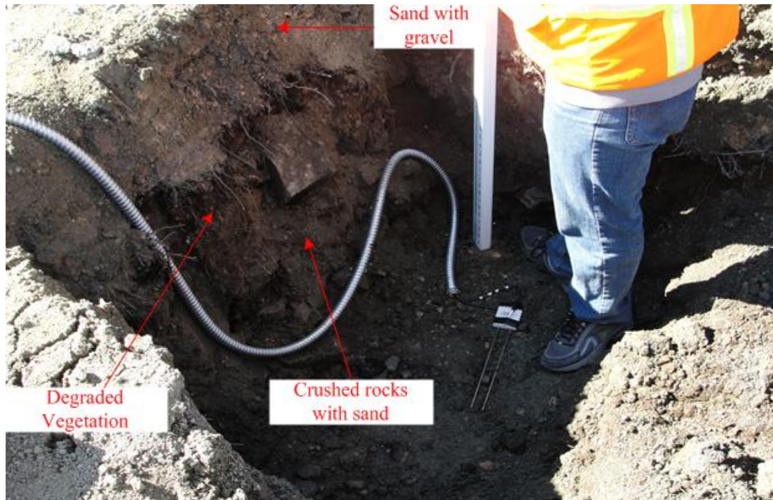
Figure 23. Excavation pit at the center of the road for sensor 13
