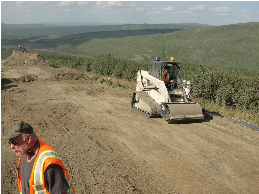
Figure 28. Compaction of the backfilled soils
