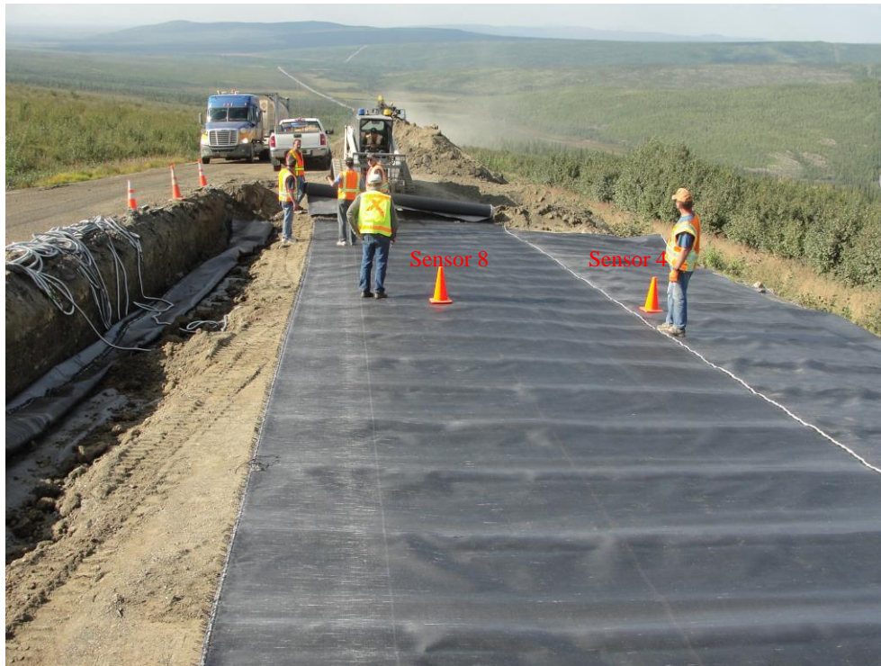
Figure 29. Installation of the second layer of wicking fabric
