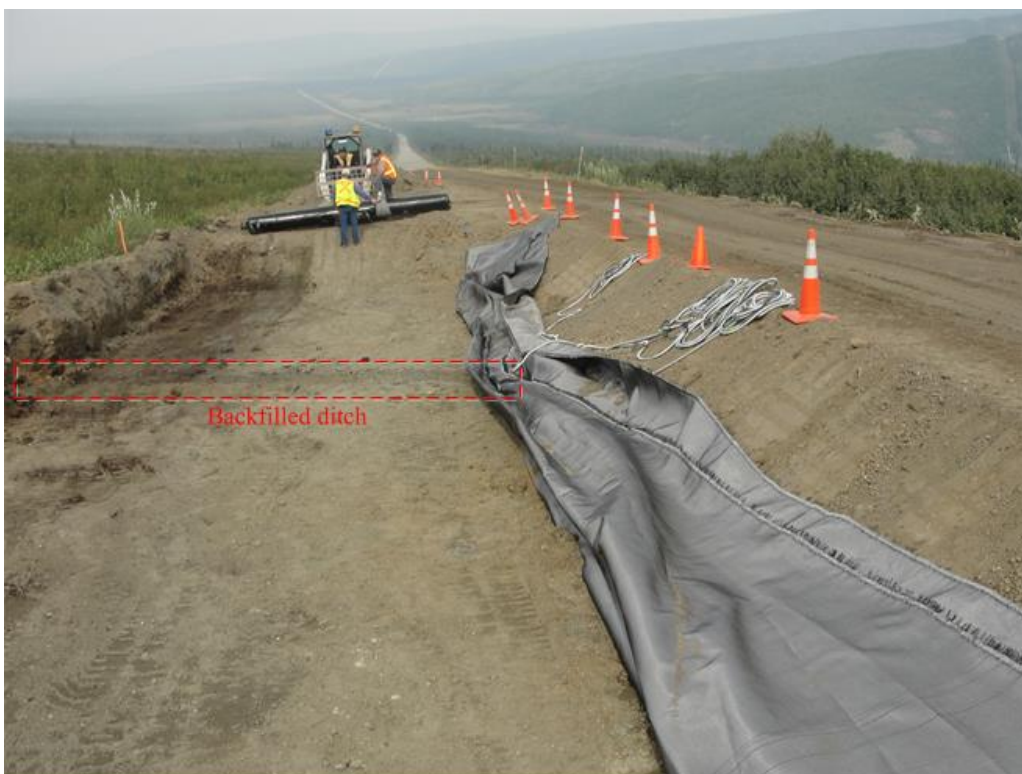
Figure 36. After installation of sensors 16, 19, and 22
