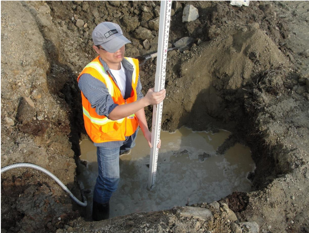
Figure 34. Installation of sensor 20
