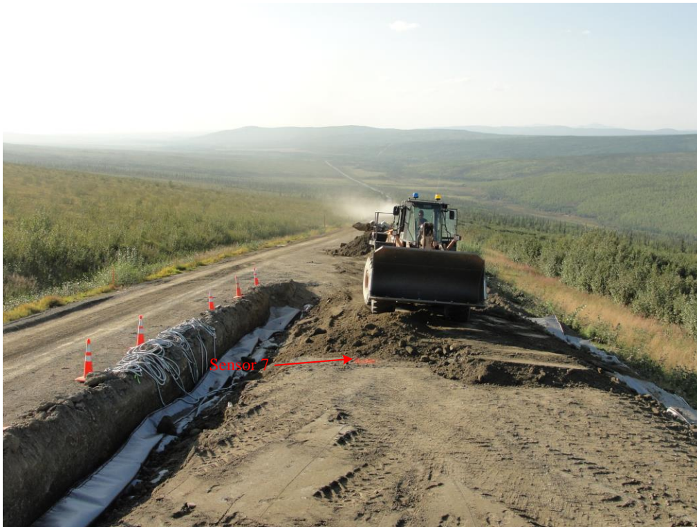
Figure 30. Installation of sensors 3 and 7 and backfill the excavation
