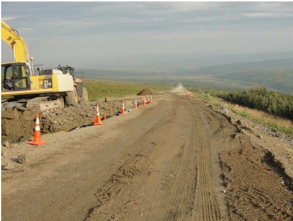
Figure 31. The lane on the east half of the road after construction
