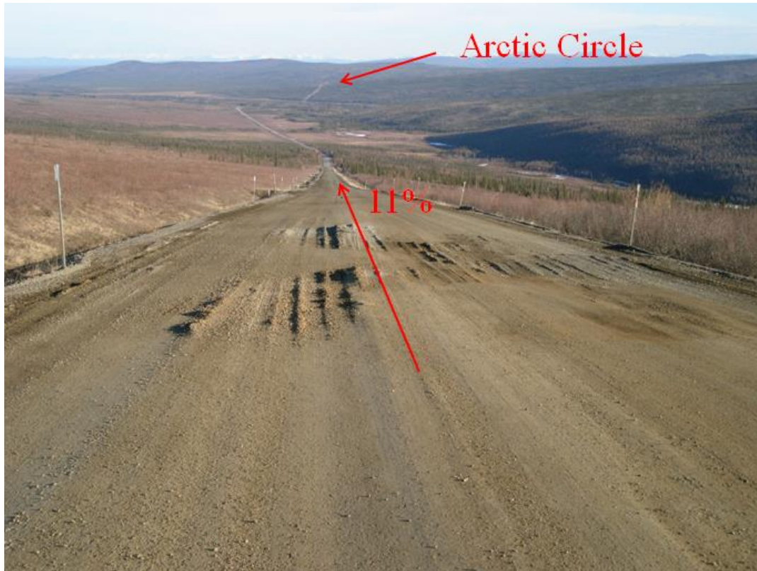
Figure 2. Frost boils at Beaver Slide on May 12, 2012 (looking north)
