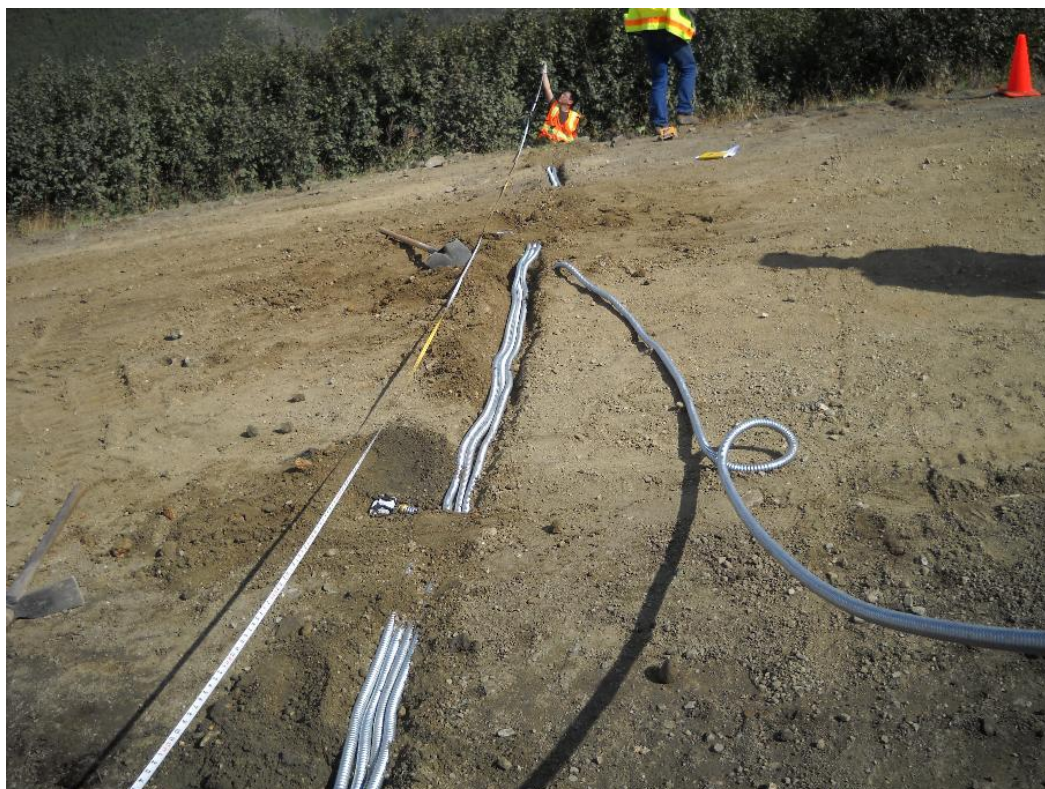
Figure 25. Installation of the aluminum conduits
