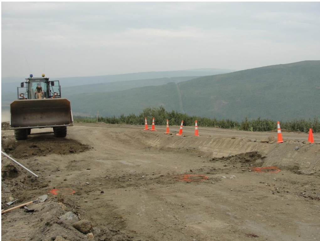
Figure 41. Installation of sensors 10, 14, and 17
