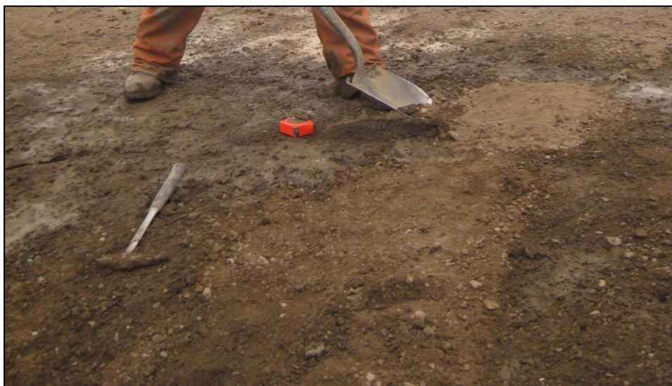
Figure 3.9. The backfilled location of TH09-1403 (to the right of the spade), and the backfilled trench.
