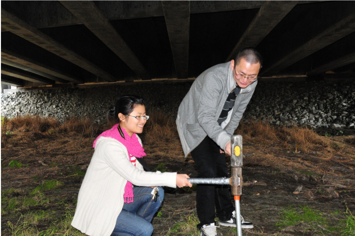
Figure 2.1 Installation of a temperature monitoring conduct at the Campbell Creek bridge site.
