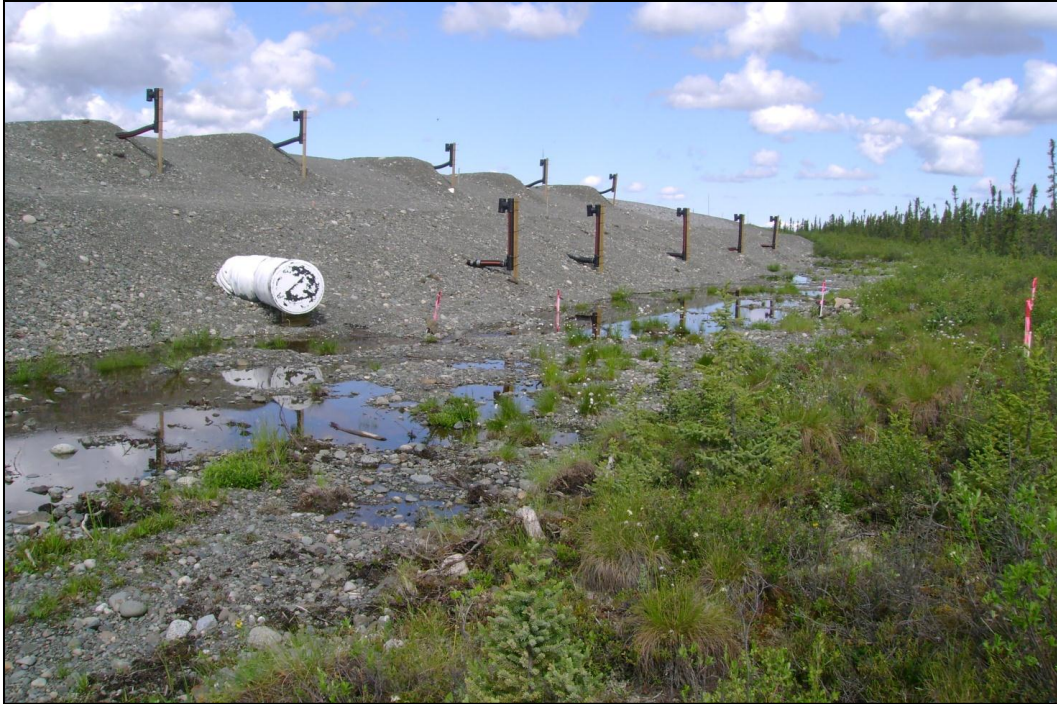
Figure 1. Water ponding on the uphill side of the Alaska Highway embankment, near Beaver Creek, Yukon, Canada. (Photography courtesy of D. Fortier)
