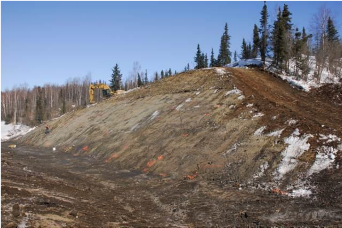
Figure 4.1 Cut slope at Dalton Highway 9 Mile Hill construction project location
