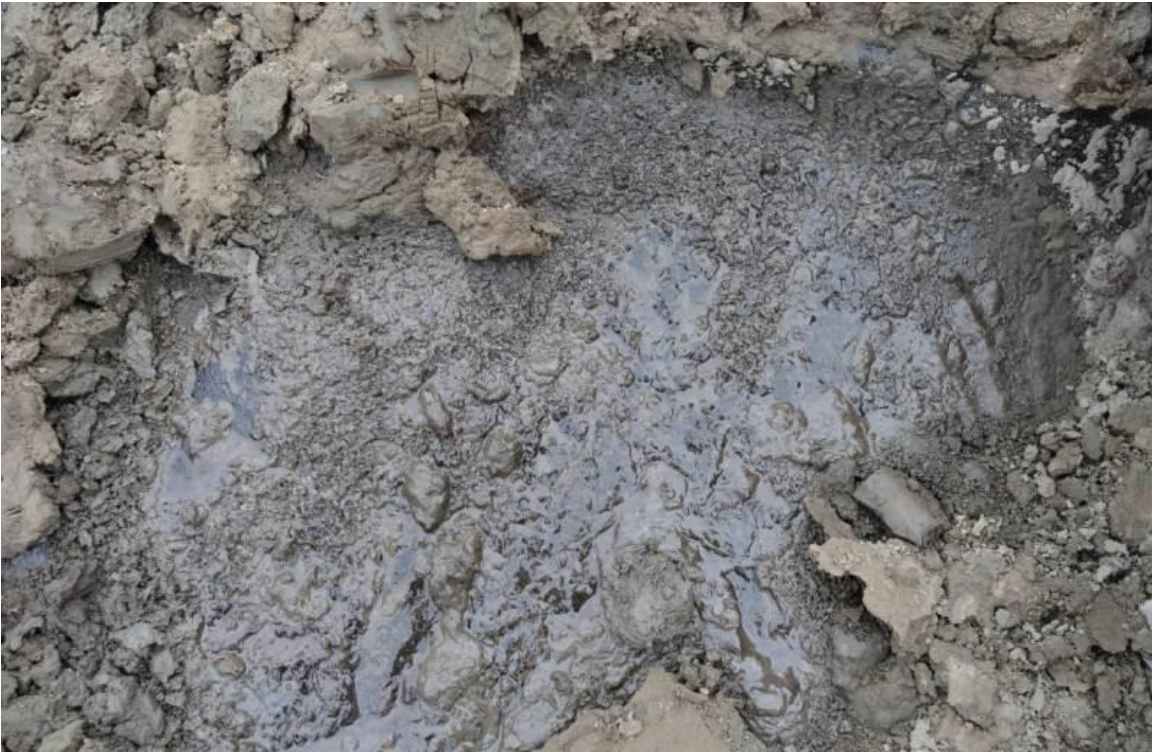
Figure 4.9 Ice exposed in the cut slope
