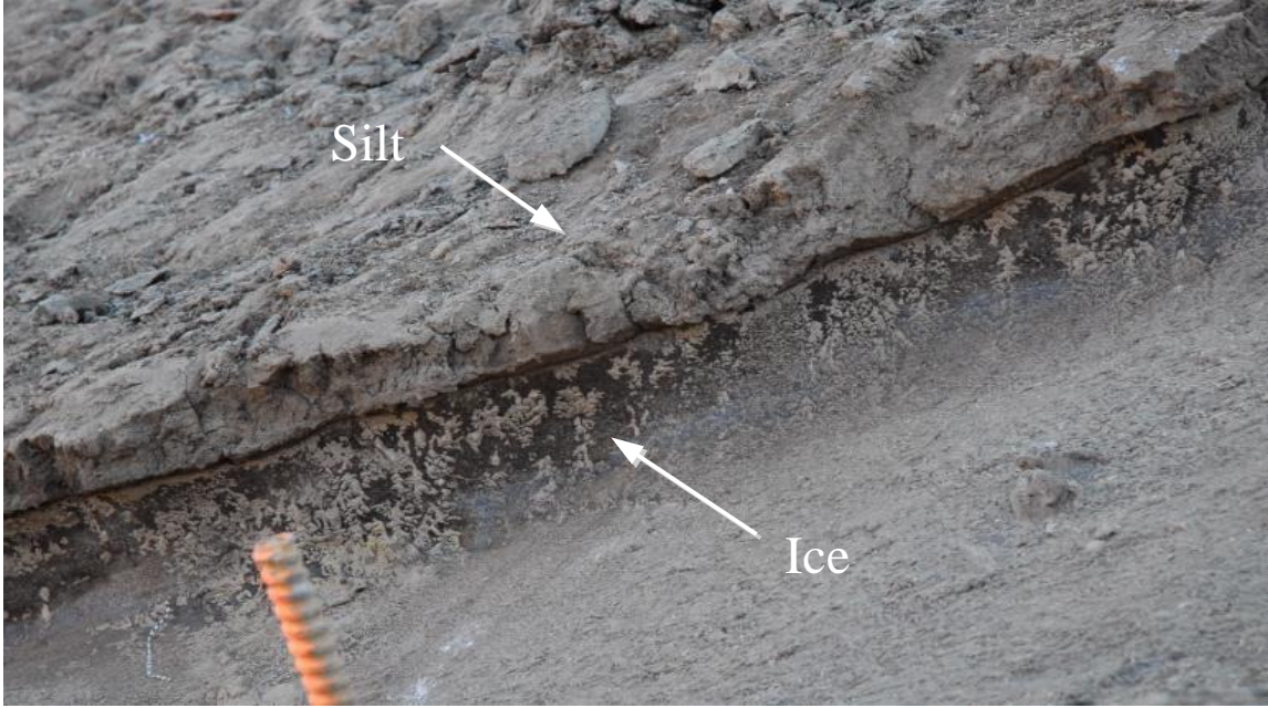
Figure 4.8 Ice in the cut slope
