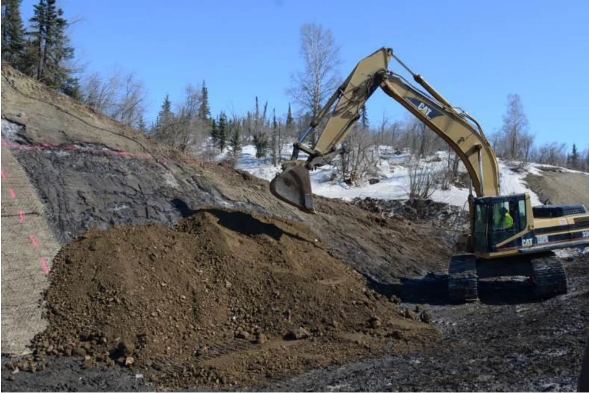
Figure 4.24 Construction of Section D
