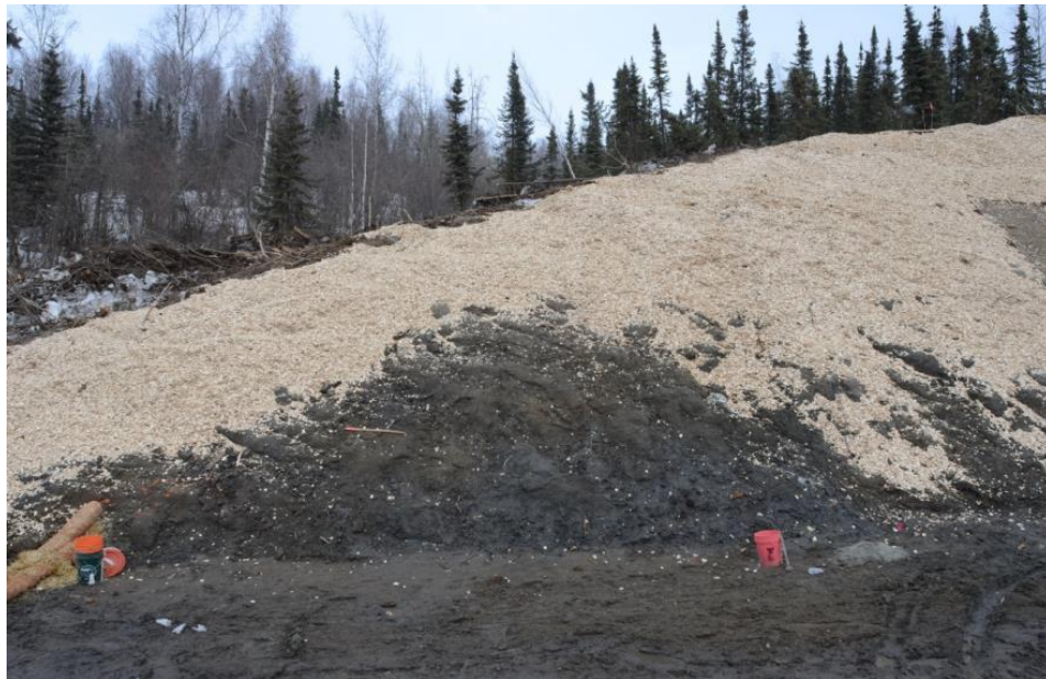
Figure 7.24 Section A after construction on April 26, 2013
