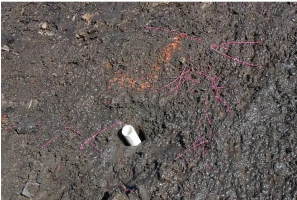
Figure 4.6 Instrumentation hole with sensor housing installed
