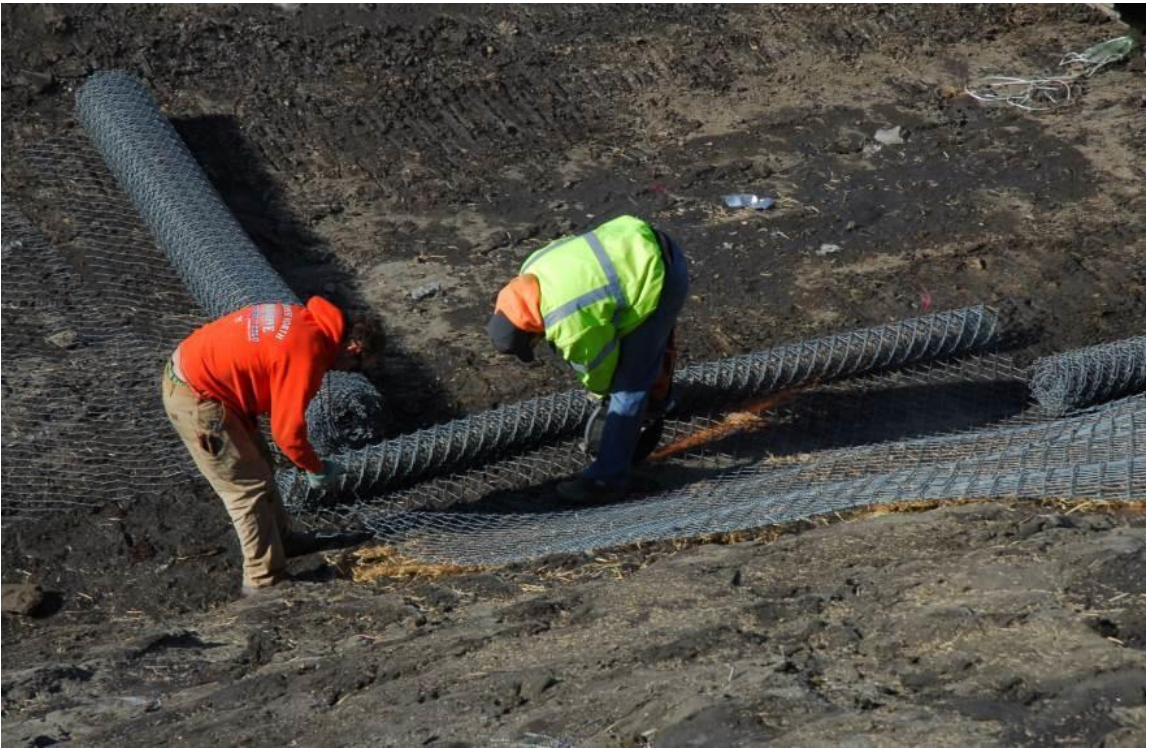
Figure 4.20 Cutting away excess Tecco-mesh
