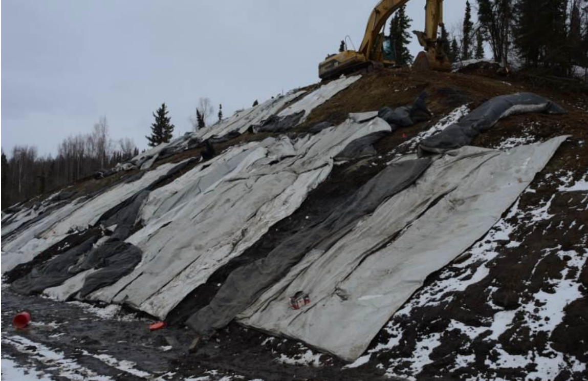
Figure 4.10 Cut slope protected from erosion during drilling
