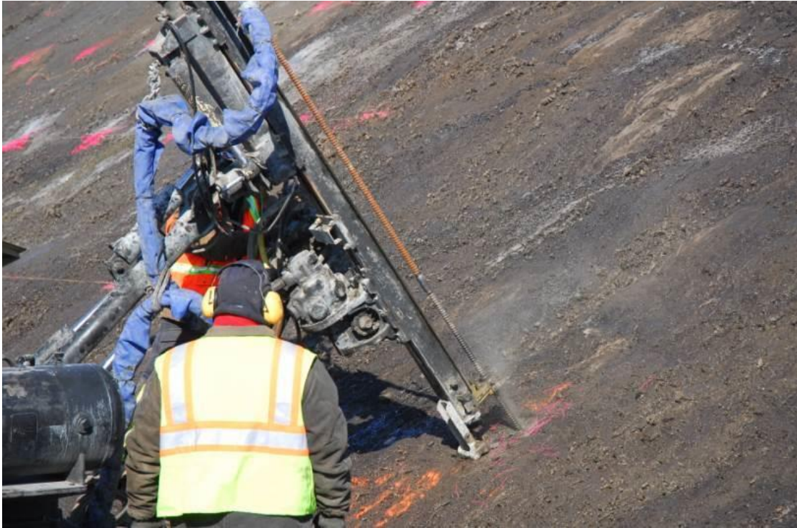
Figure 4.3 Drilling on the cut slope
