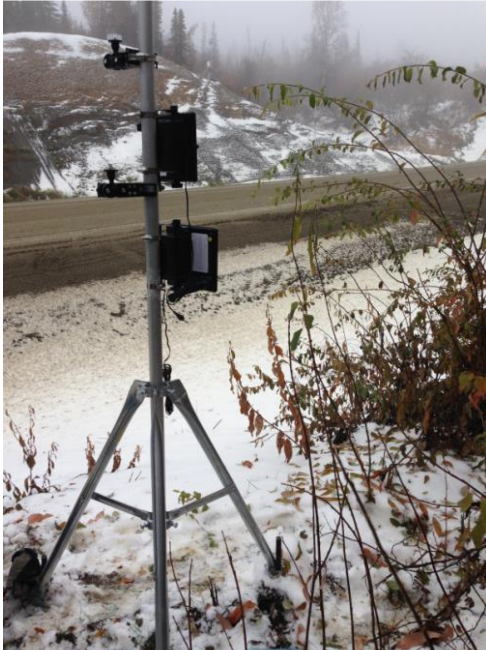
Figure 5.11 Two cameras installed for slope monitoring
