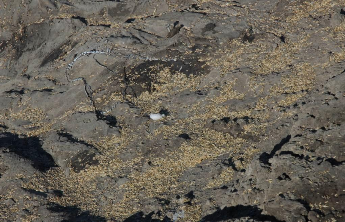
Figure 4.14 Seeded cut slope
