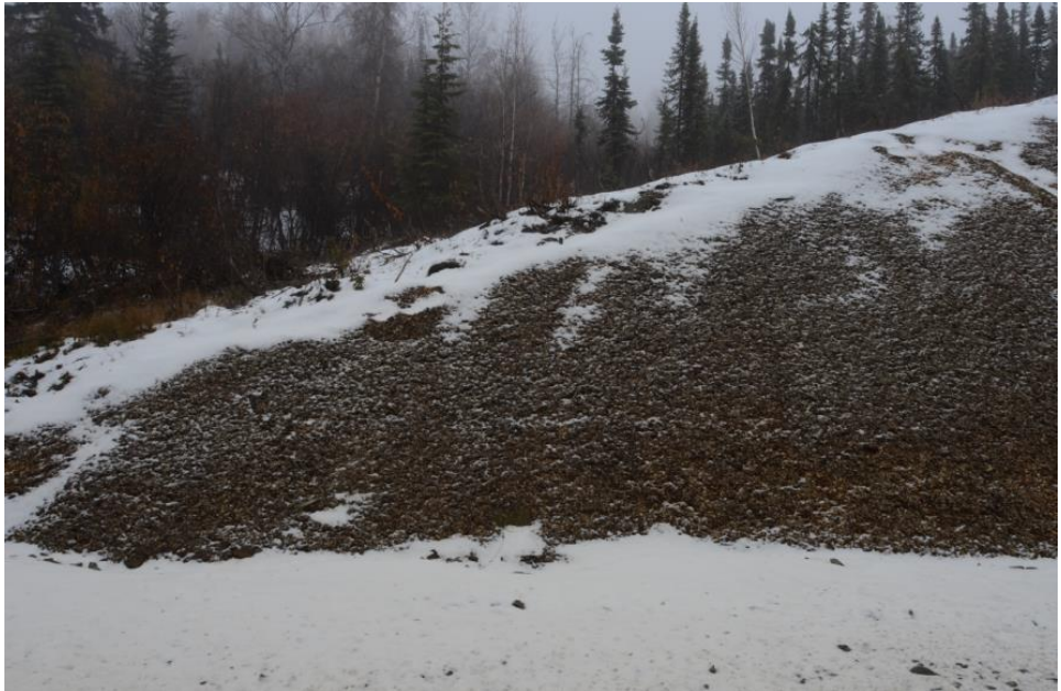
Figure 7.26 Section A with more wood chips on September 27, 2013
