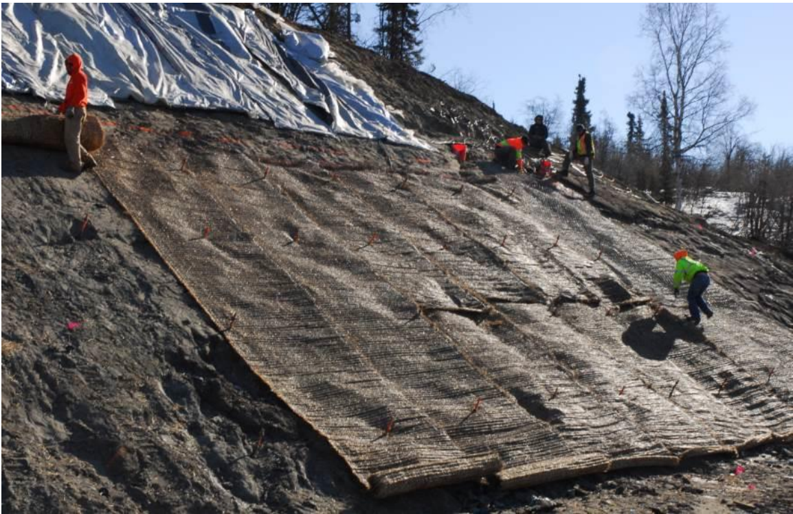
Figure 4.16 Placement of coconut erosion control matting
