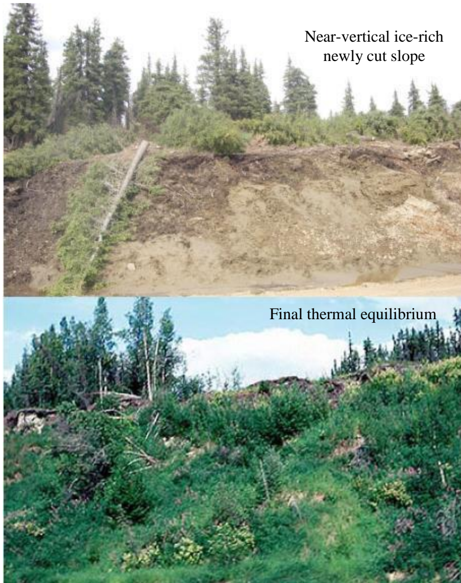
Figure 2.1 Ice-rich cut slope (Mageau and Rooney, 1984)
