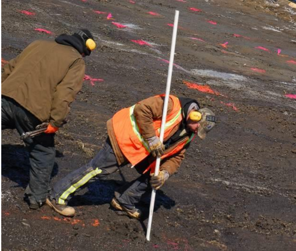
Figure 4.5 Installation for sensor housing
