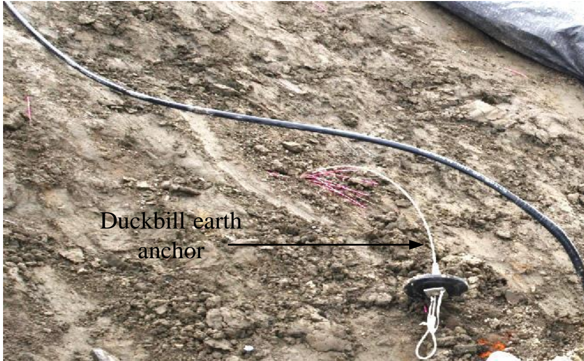
Figure 4.11 Cable end of installed duckbill earth anchor
