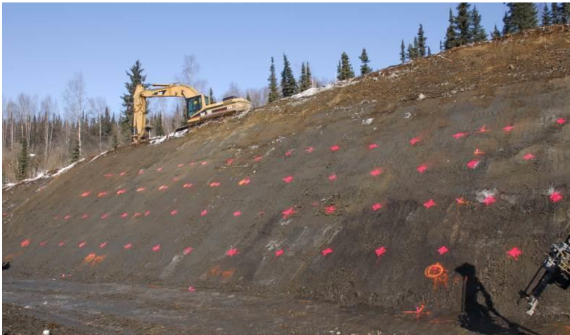
Figure 4.2 Layout on the cut slope
