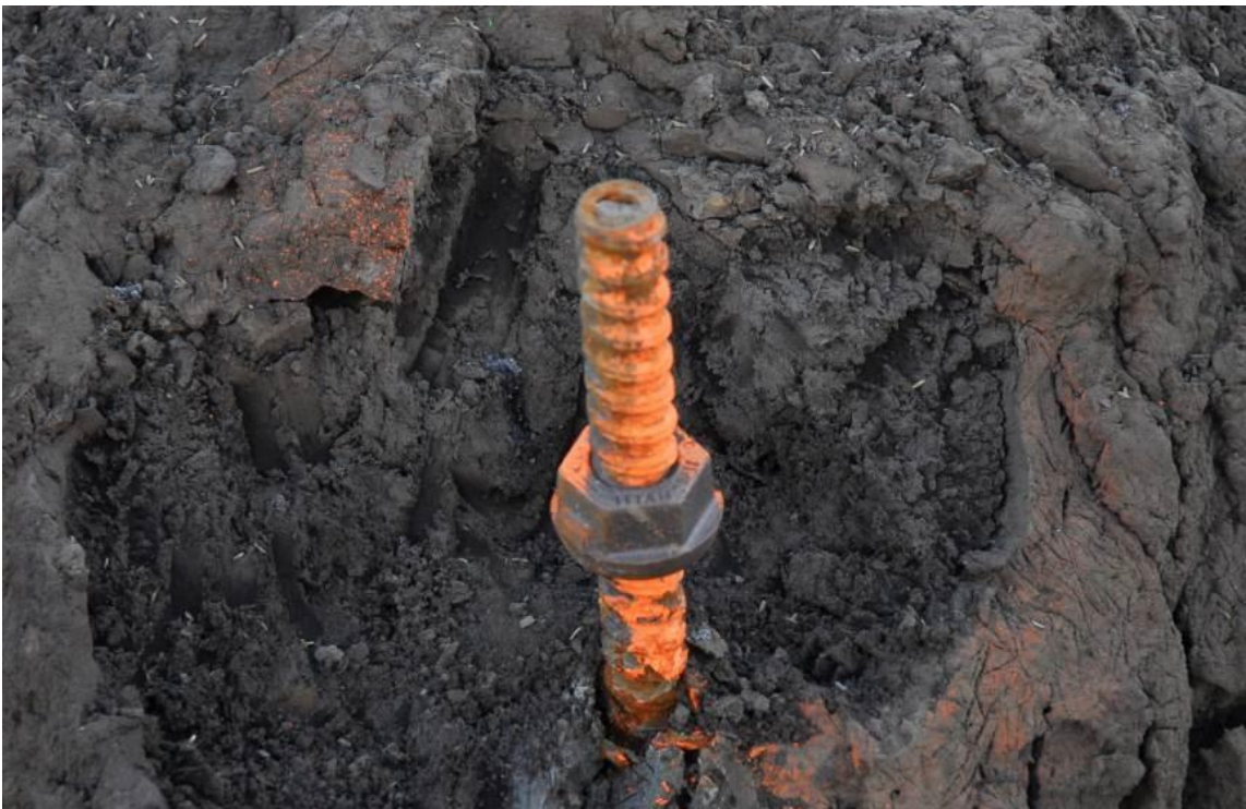
Figure 4.12 Installation of hollow rebar anchor
