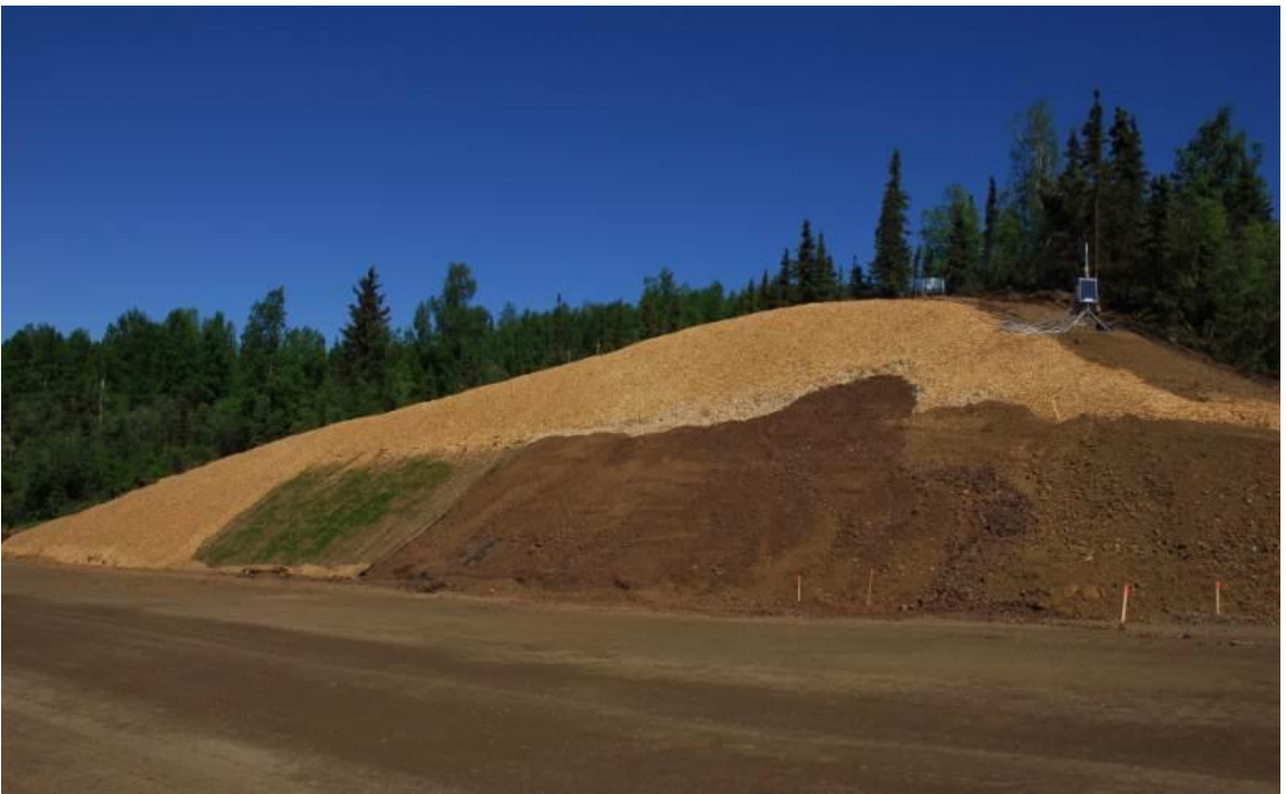
Figure 6.8 Cut slope after construction on Section C
