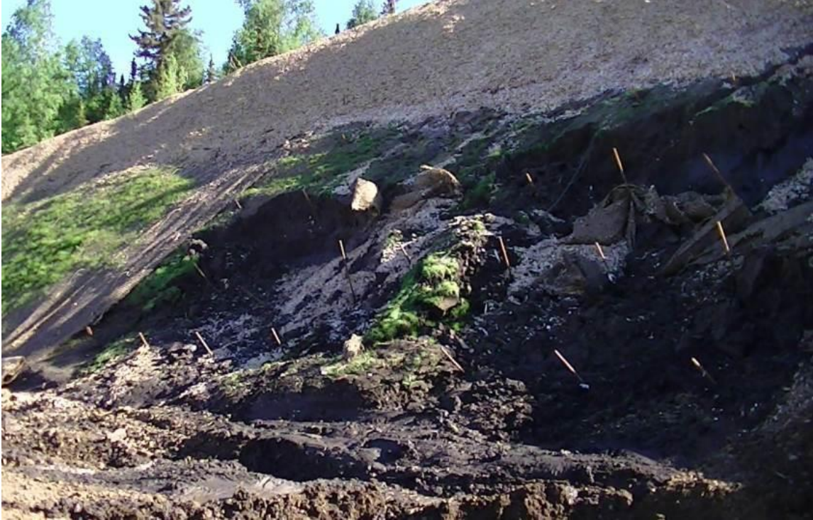
Figure 6.5 Section C without Tecco-mesh and coconut blanket
