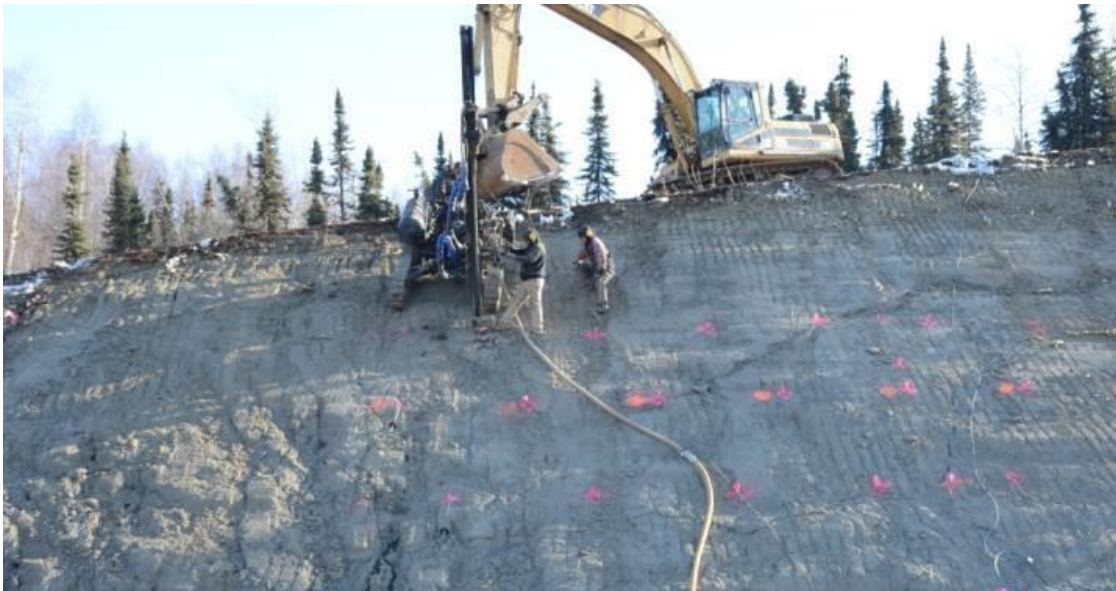
Figure 4.4 Drilling at the upper part of the slope
