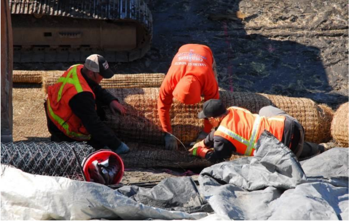
Figure 4.15 Placement of the coconut erosion control matting
