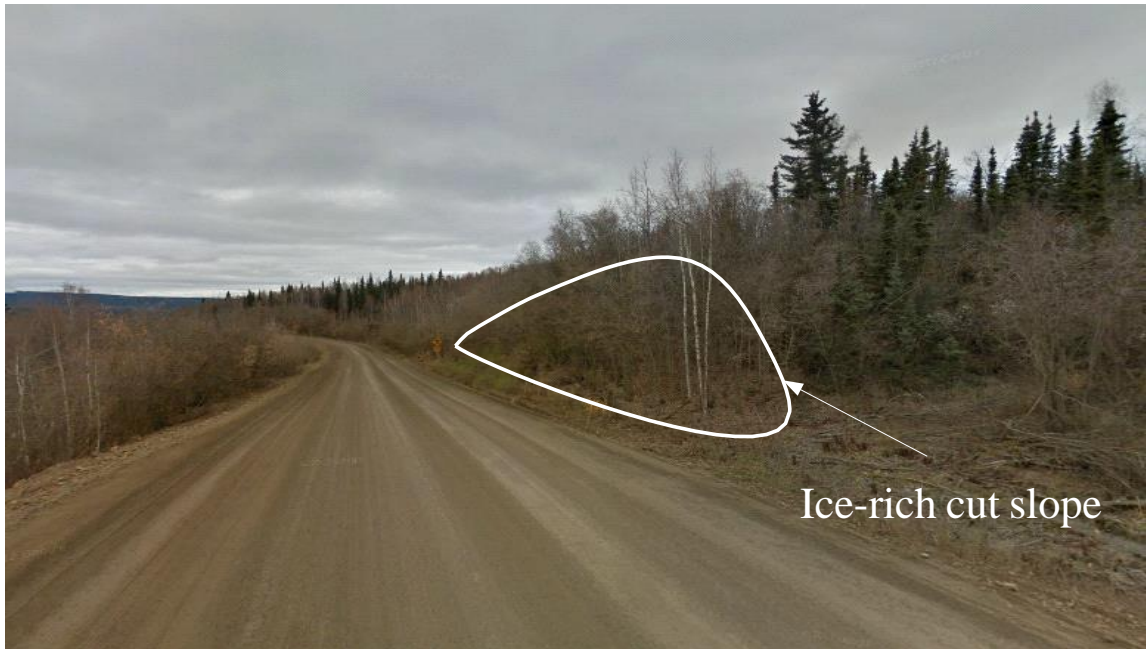
Figure 1.4 Ice-rich cut slope site prior to construction (looking north)
