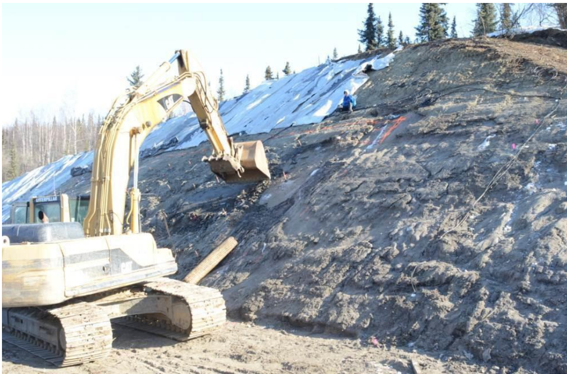
Figure 4.13 Re-smoothing the cut slope surface
