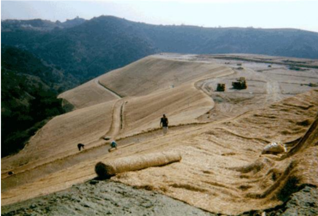
Figure 2.4 Erosion control blanket (from http://www.thelandstewards.com/blankets.htm )
