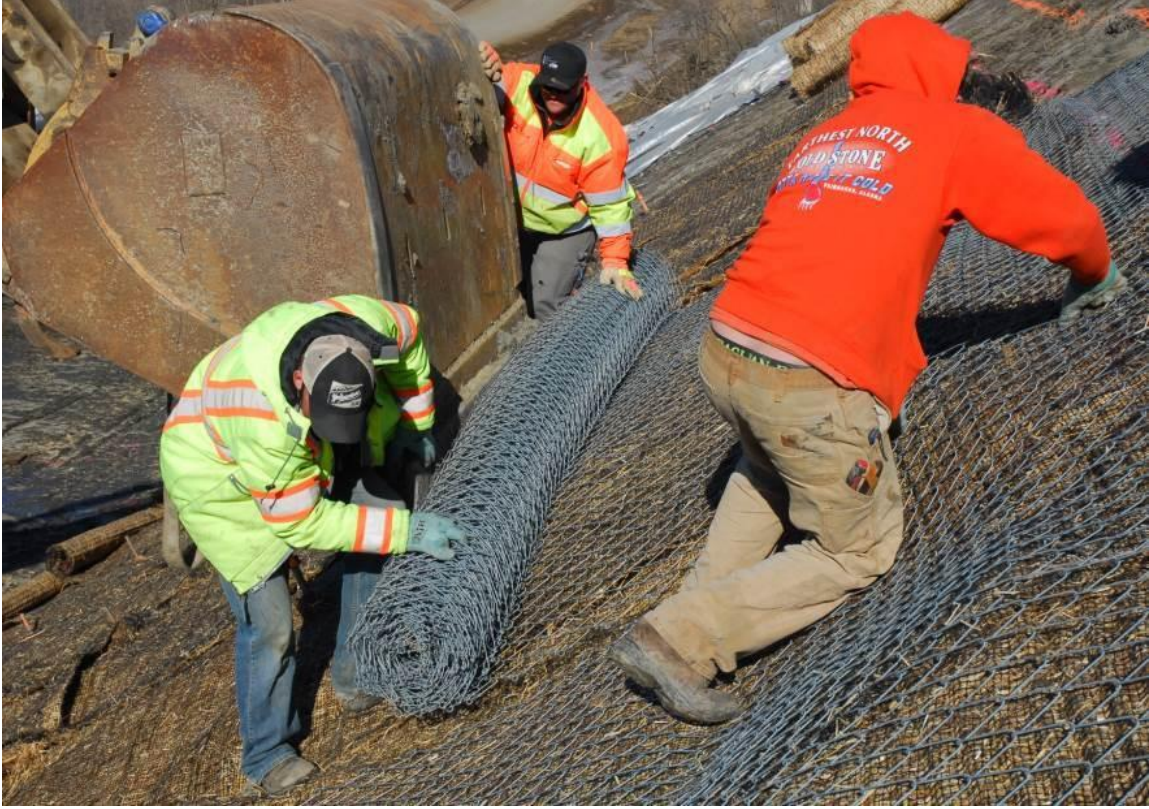
Figure 4.19 Placement of Tecco-mesh
