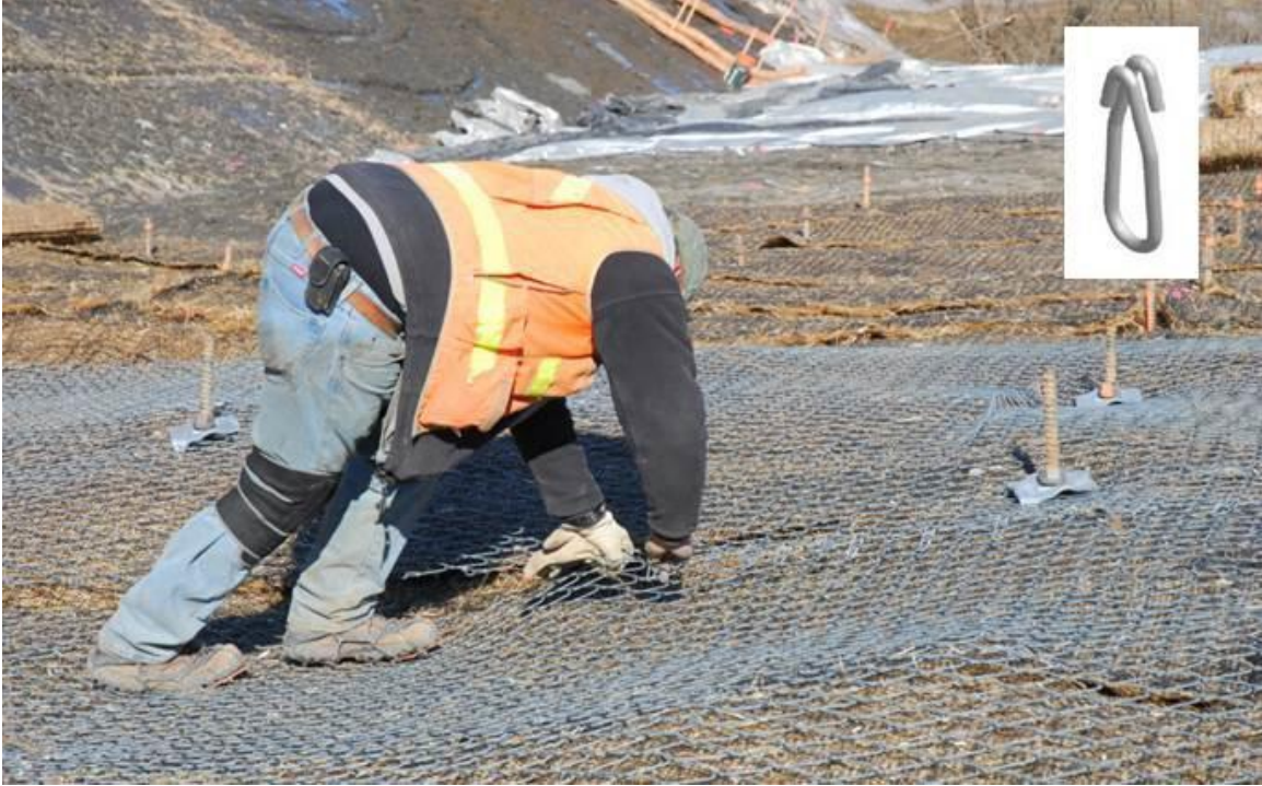
Figure 4.21 Connecting adjacent Tecco-mesh strips
