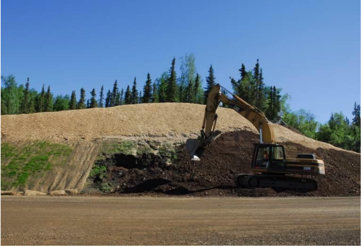
Figure 6.7 Covering Section C with crushed rock
