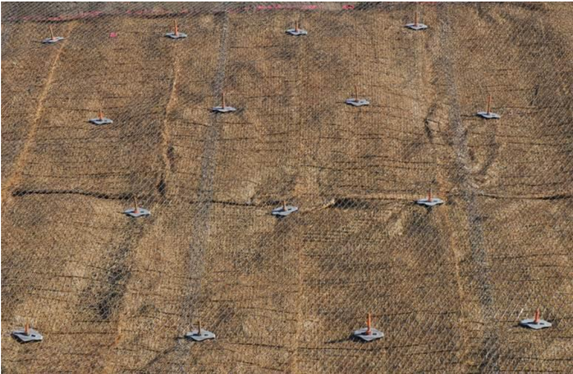
Figure 4.22 Section C appearance after construction
