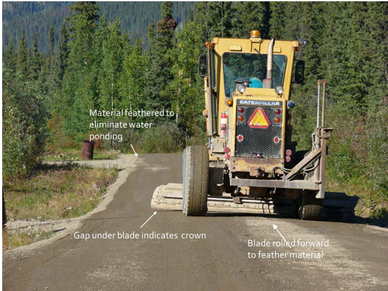
Figure 4.10 Proper grading improves roadway performance
