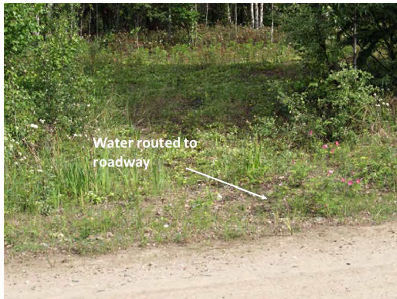
Figure 4.9 Water routed to roadway due to improper ditching
