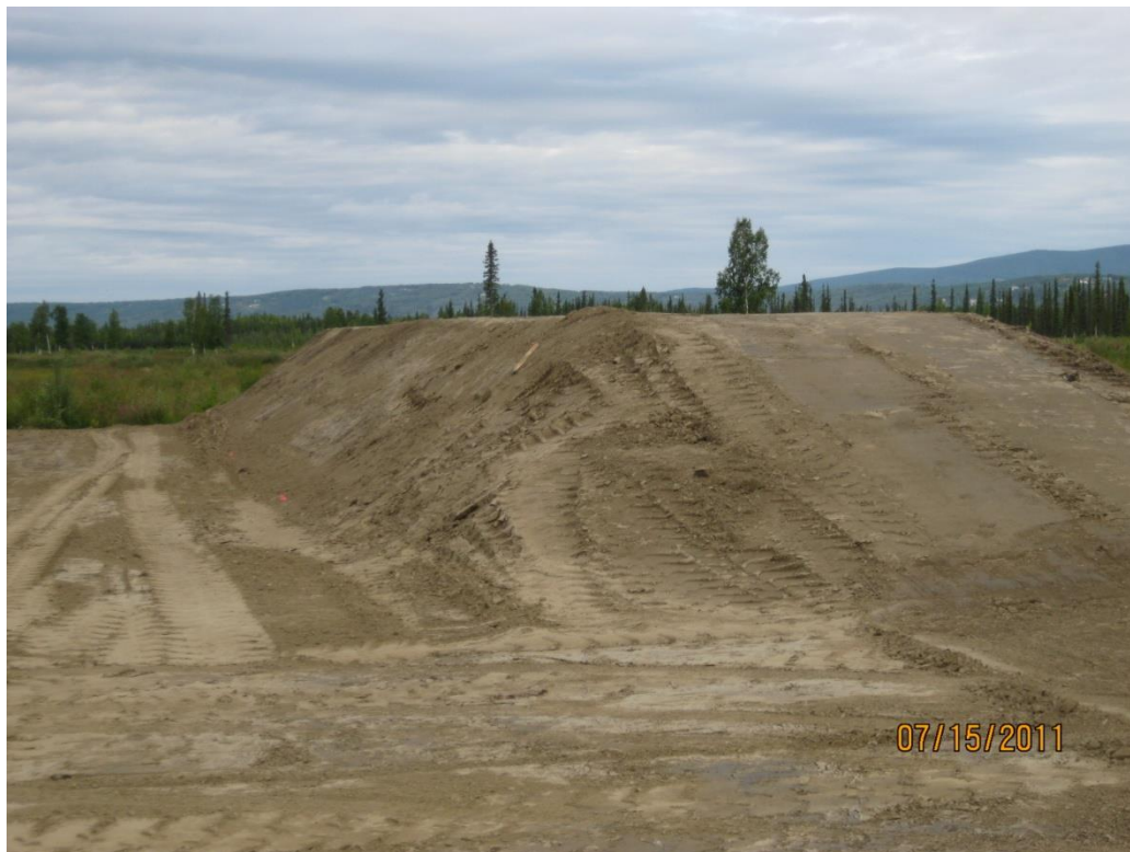
Fig. 3-6: Embankment prior to installation of test strips
