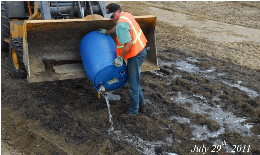
Fig. 3-9: Addition of liquid additive
