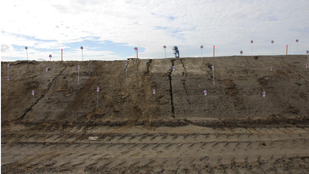
Fig. 3-8: Embankment before treatment (north slope)
