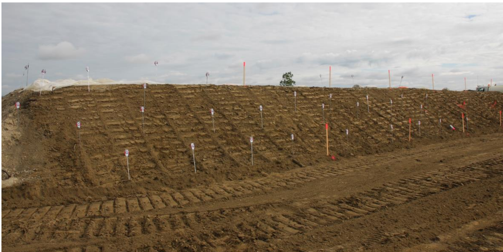
Fig. 3-7: Embankment compaction before treatment (south slope)
