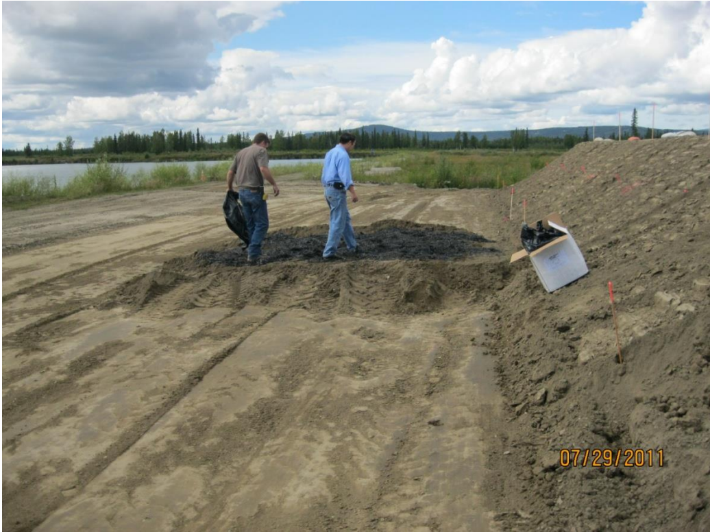
Fig. 3-10: Geofibers added to stockpiled soil
