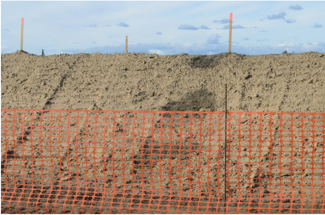
Fig. 3-14: Slope after hydroseeding
