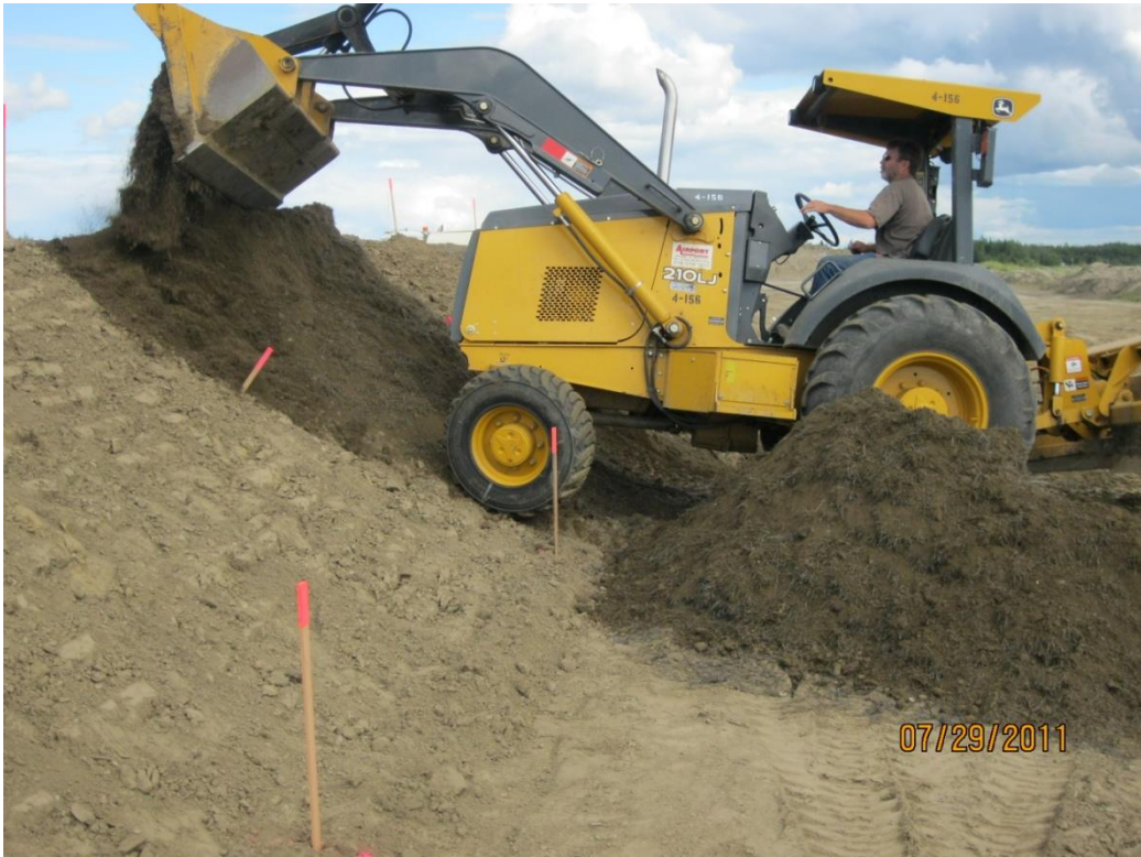
Fig. 3-12: Treated soil pushed onto side of slope
