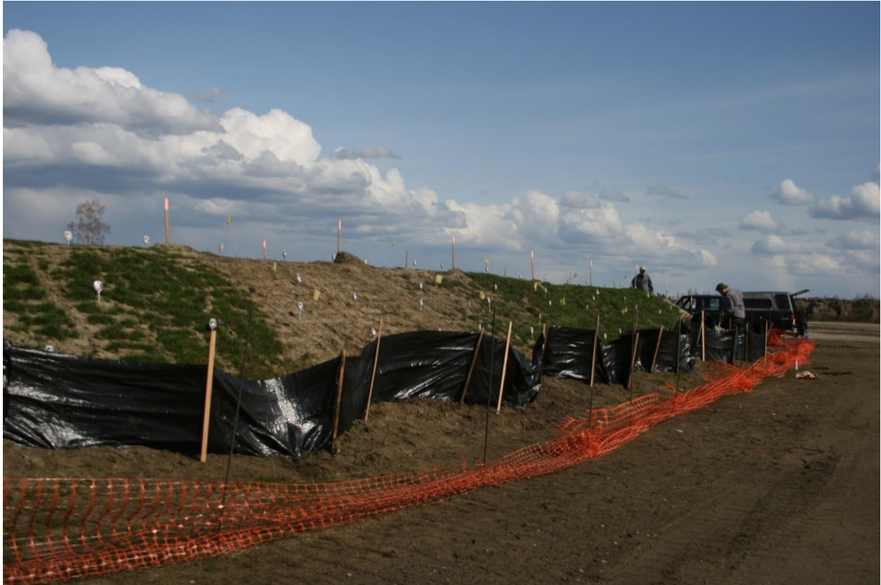
Fig. 3-17: Installed silt fence
