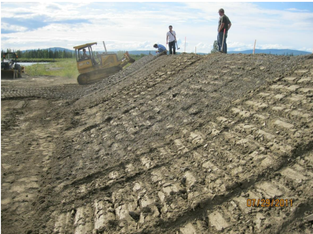
Fig. 3-13: Bulldozer running over side of slope to provide compaction
