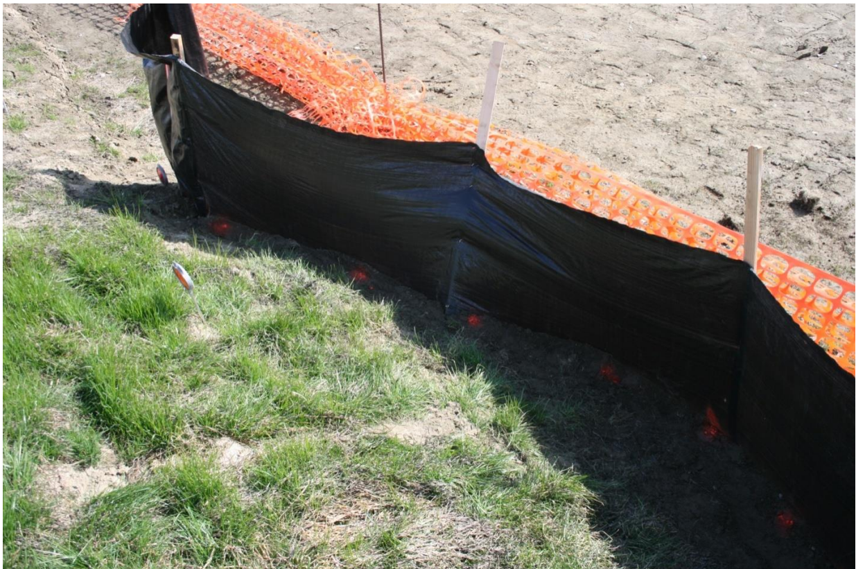
Fig. 3-18: Dots painted below base of silt fence allow for identification of runoff material from the slope
