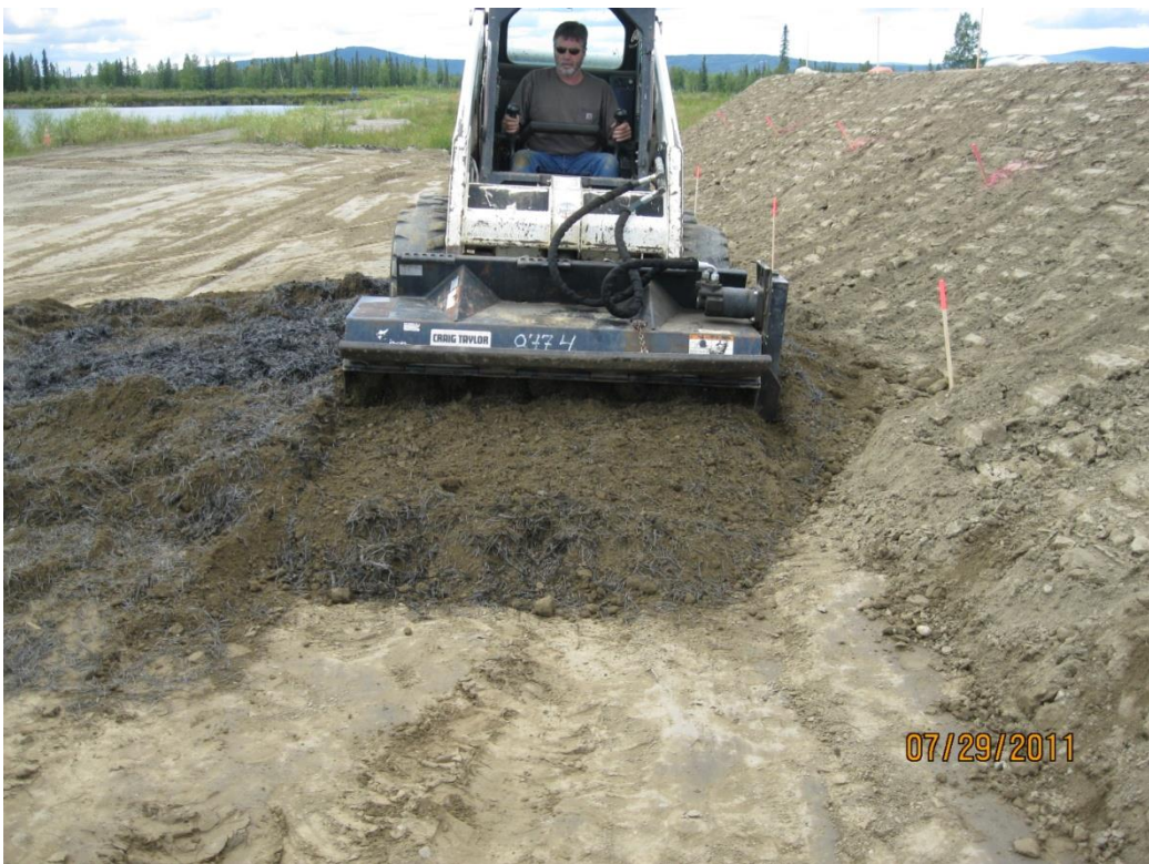
Fig. 3-11: Rototiller blending geofibers with stockpiled soils
