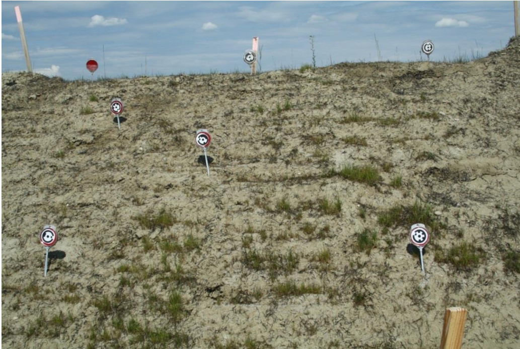
Fig. 4-3: Geofibers + EnviroKleen treatment for erosion control (photo taken June 22, 2012)
