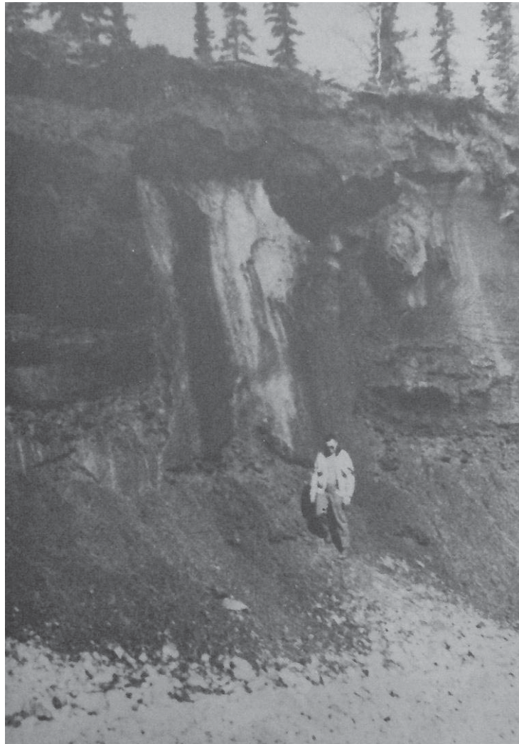
Figure 4.1. Ice wedge exposed during construction of the pipeline haul road near Hess Creek (Andersland & Anderson 1978).
