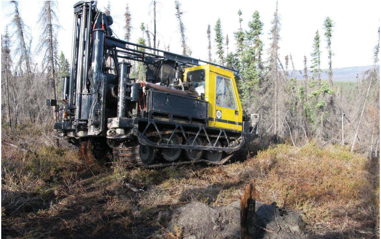
Figure 2.1. Drill rig at the Dalton Highway Innovation Project field site, May 2008.
