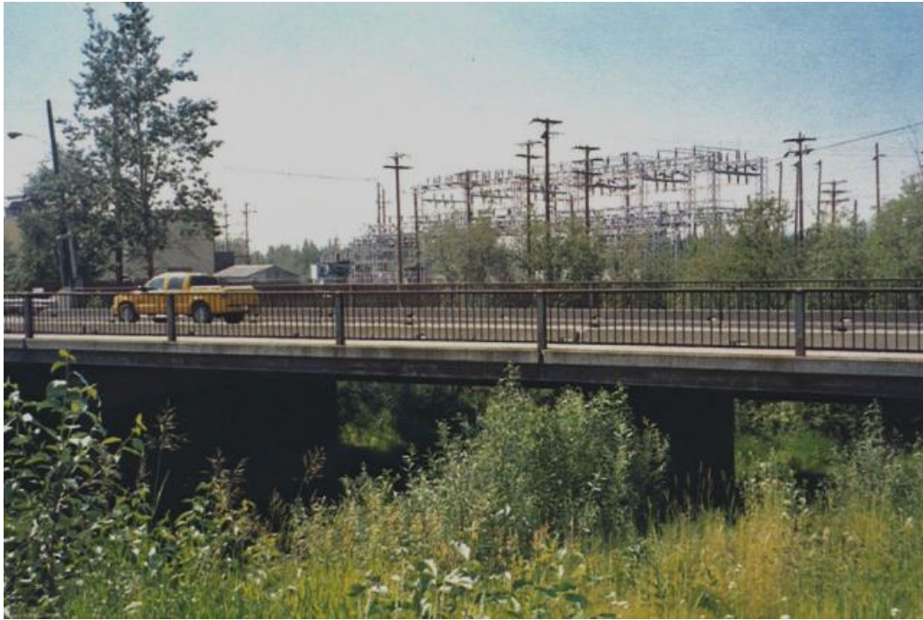
Figure 1.1 Side view of the Noyes Slough Bridge
