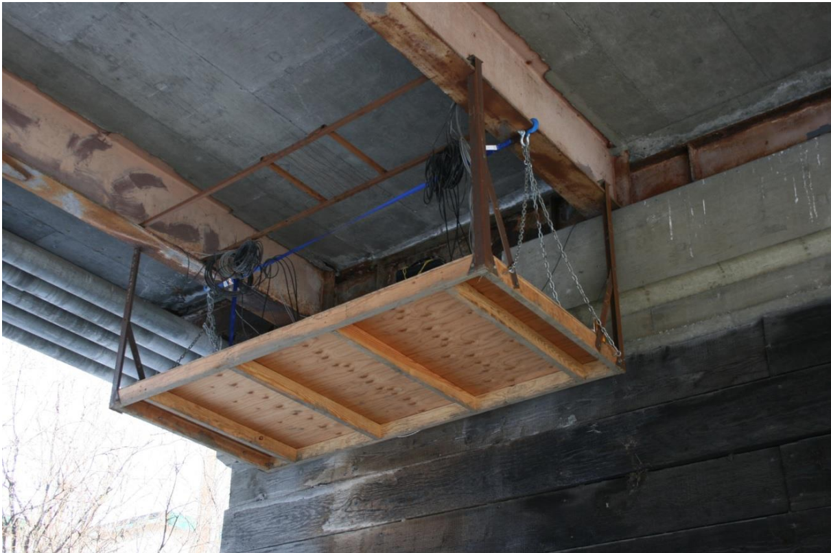
Figure 1.5 Rolling platform and data collection staging area
