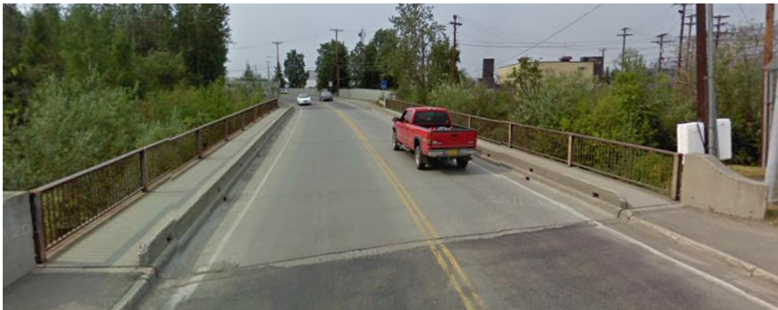
Figure 1.2 Westbound view of Noyes Slough Bridge
