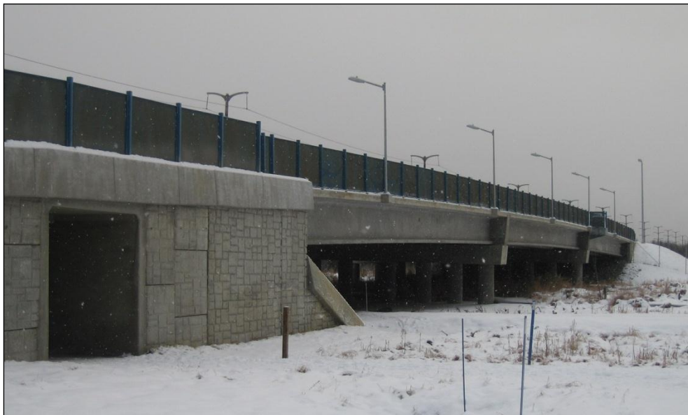
Figure 3.3: North Fork Campbell Creek Bridge.
