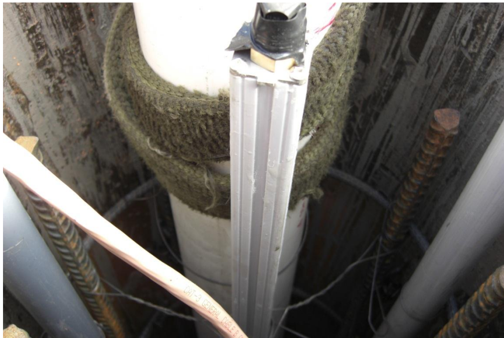
Figure 2.7: Inclinometer as installed in the test pile.
