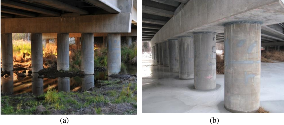
Figure 3.4: Views of the bridge substructure: (a) summer, (b) winter.
