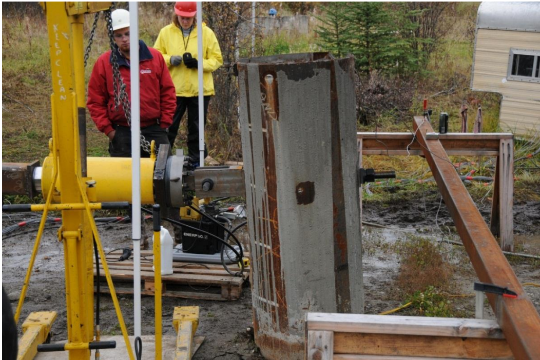
Figure 2.21: Reaction pile at final September load increment.
