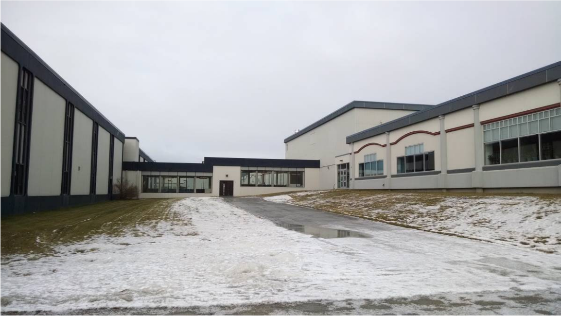
Figure 7: East High School southwest corridor doors (south and west-facing)
