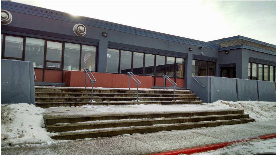
Figure 19: East High School northeast section “art wing” northwest east-facing doors
