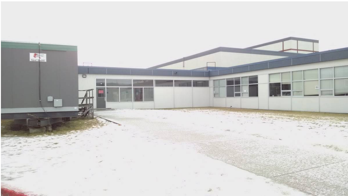
Figure 16: East High School northeast hallway north-facing door
