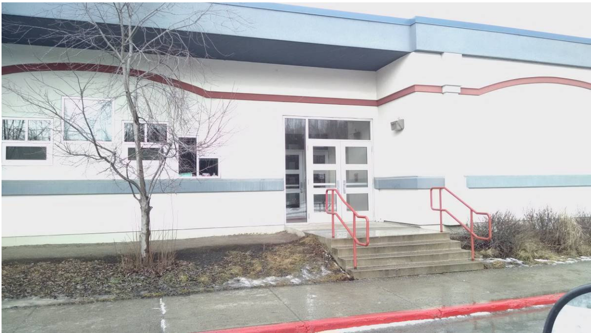
Figure 10: East High School School-Within-A-School (SWS) section southeast south-facing doors
