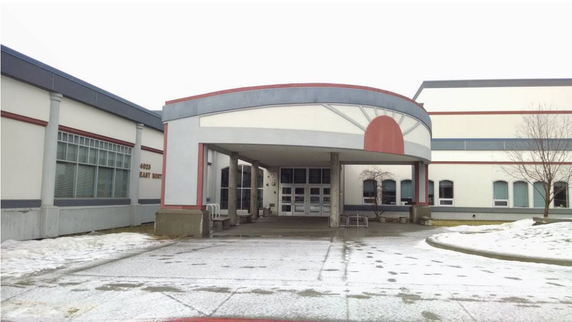
Figure 8: East High School main entrance (South)
