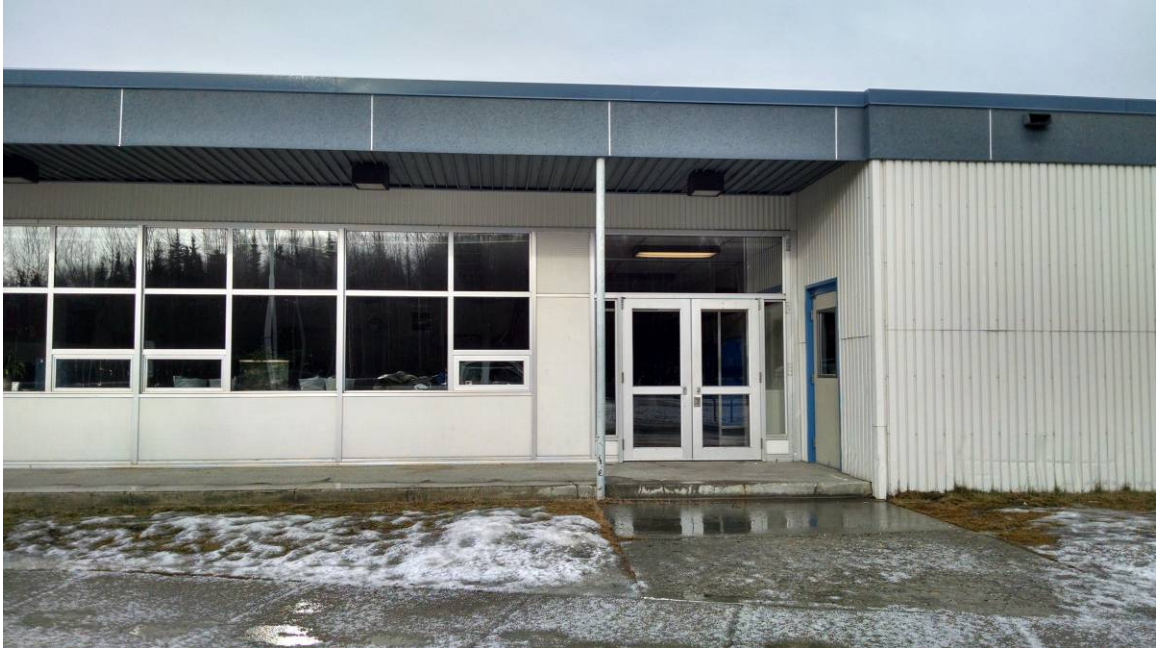
Figure 13: East High School science wing southeast south-facing doors
