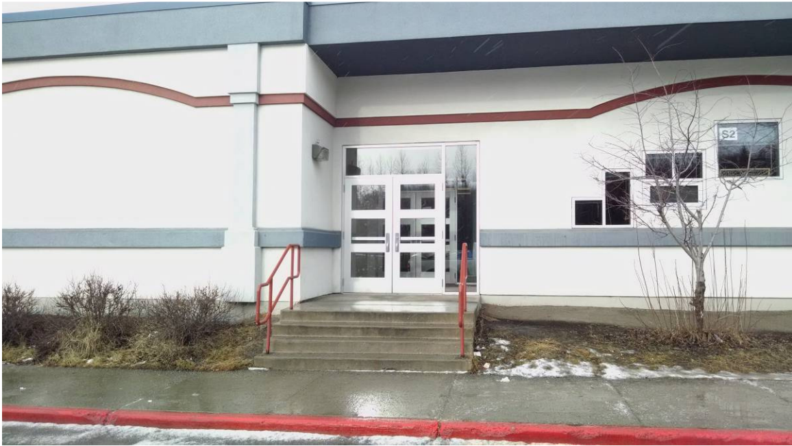
Figure 9: East High School School-Within-A-School (SWS) section southwest south facing doors
