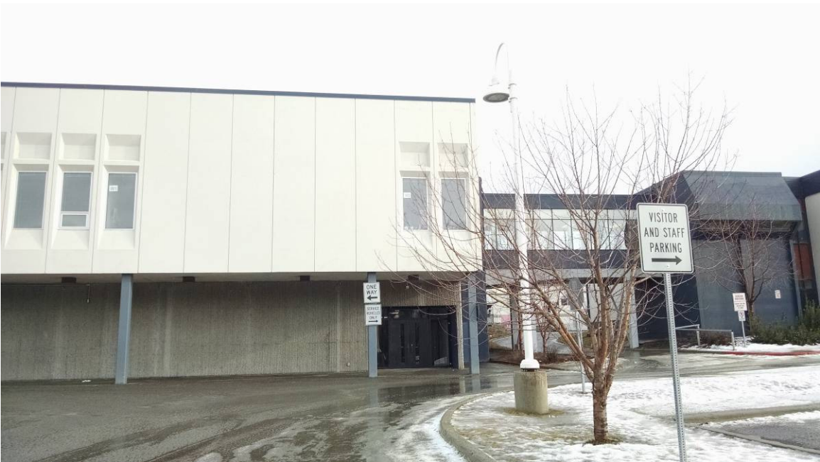
Figure 26: East High School northwest hallway west-facing doors
