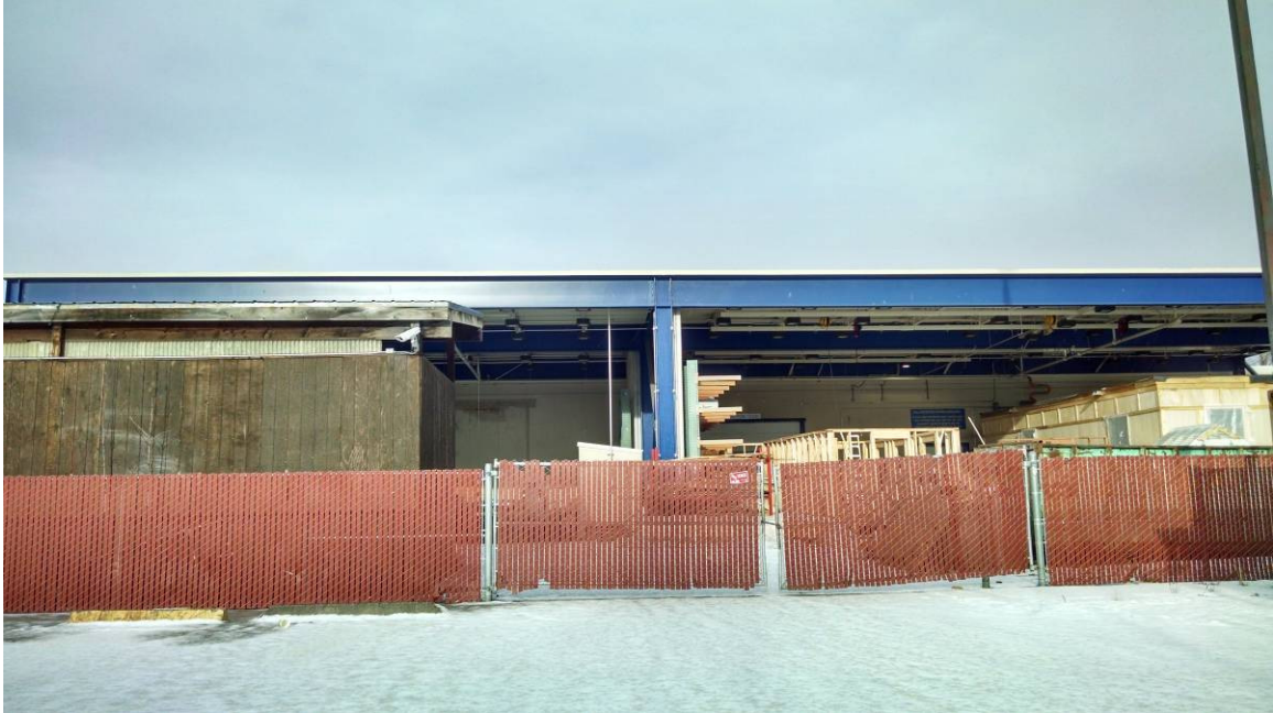
Figure 30: King Career Center South Facing Garage Doors (Southeast Portion)
