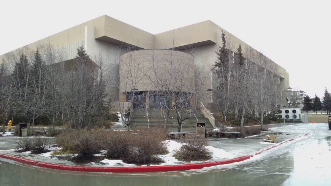
Figure 37: Sullivan Arena entrance (Southeast)
