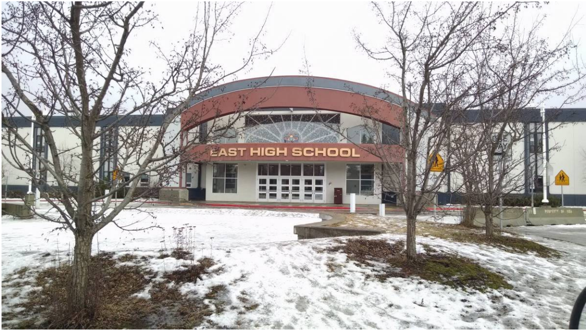
Figure 5: East High School main entrance (West)
