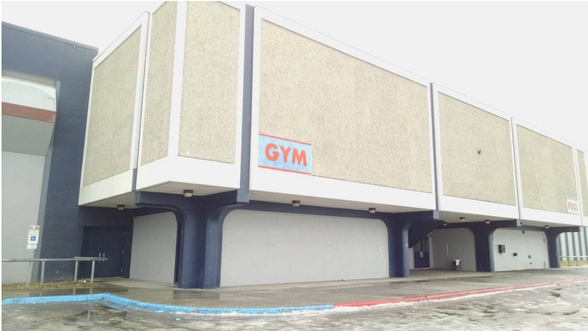
Figure 23: East High School gym north-facing emergency exit doors
