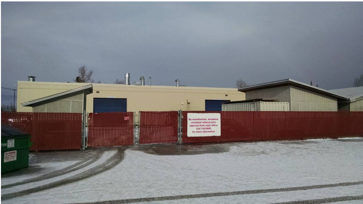
Figure 31: King Career Center South Facing Garage Doors (Southwest Portion)
