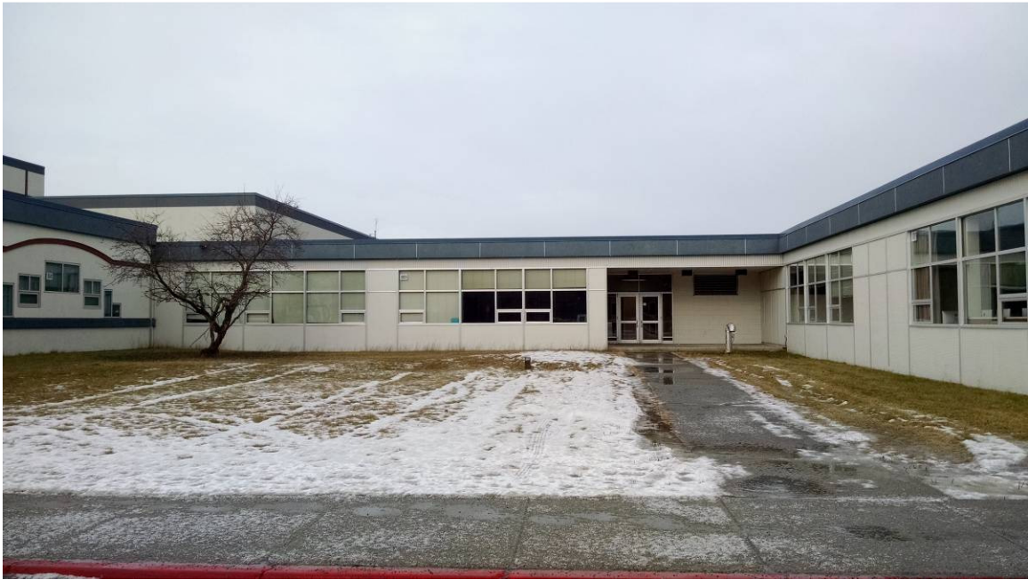
Figure 11: East High School south hallway south-facing doors
