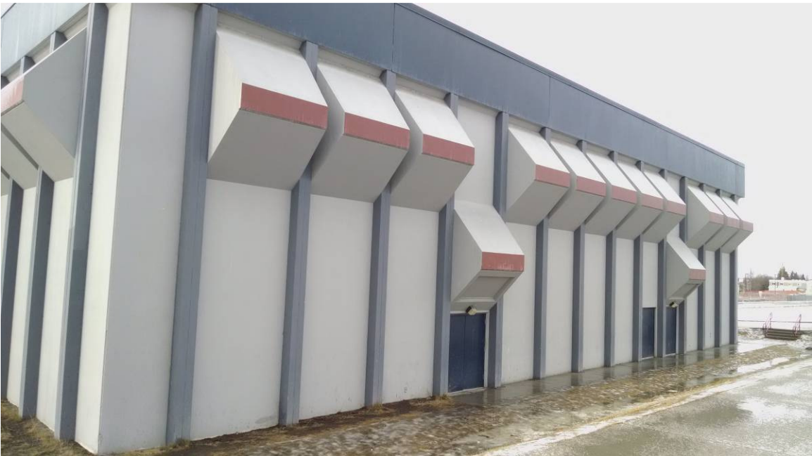
Figure 22: East High School gym west-facing emergency exit doors
