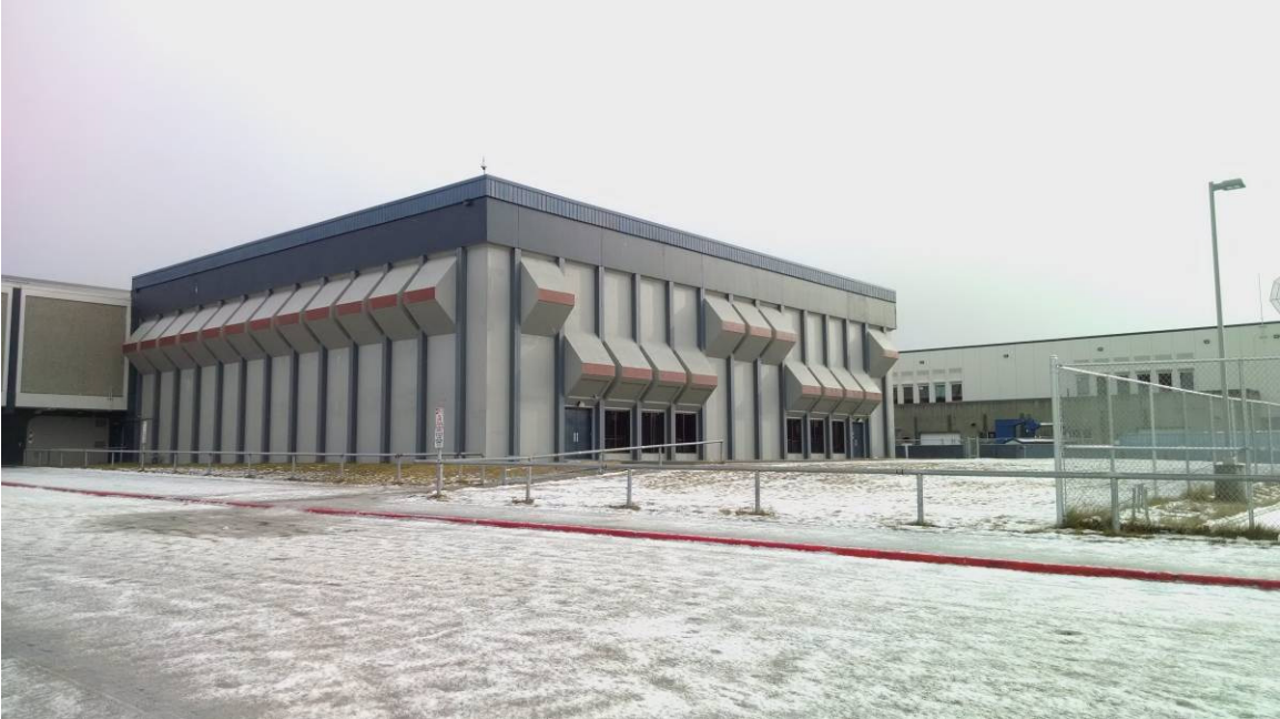
Figure 25: East High School pool doors (north and west-facing)
