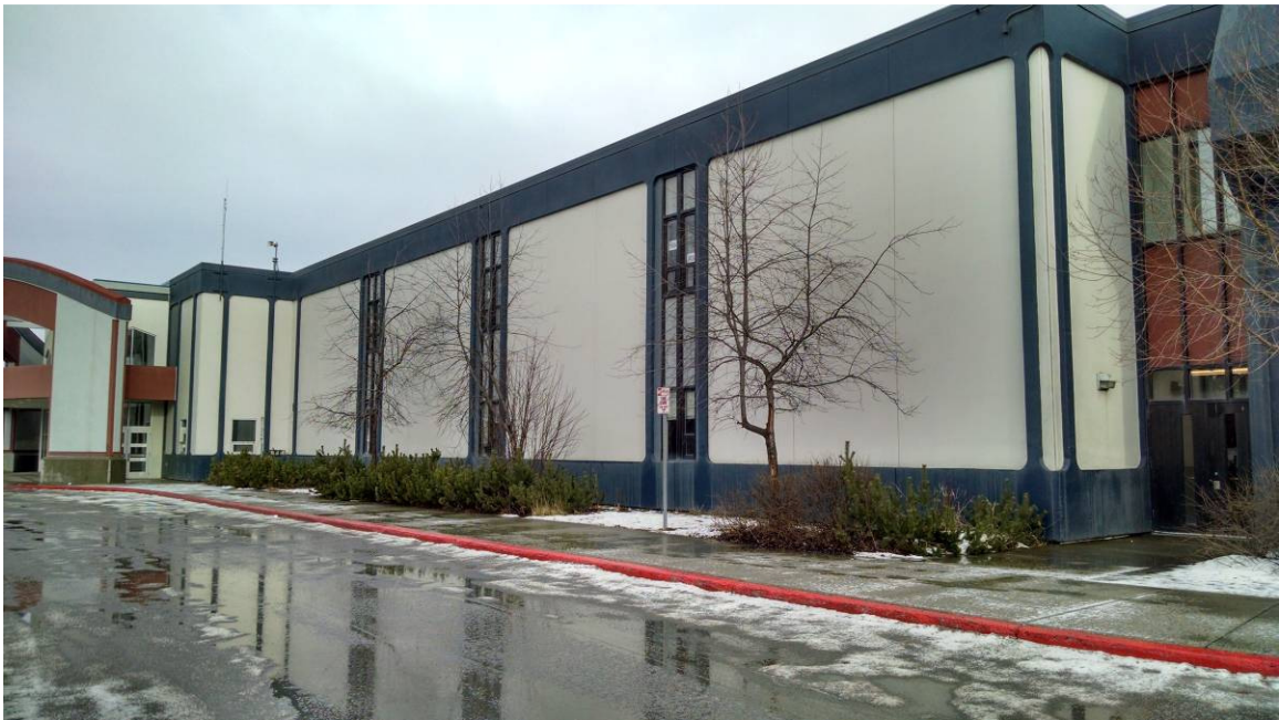
Figure 6: East High School southwest doors (south and west-facing)
