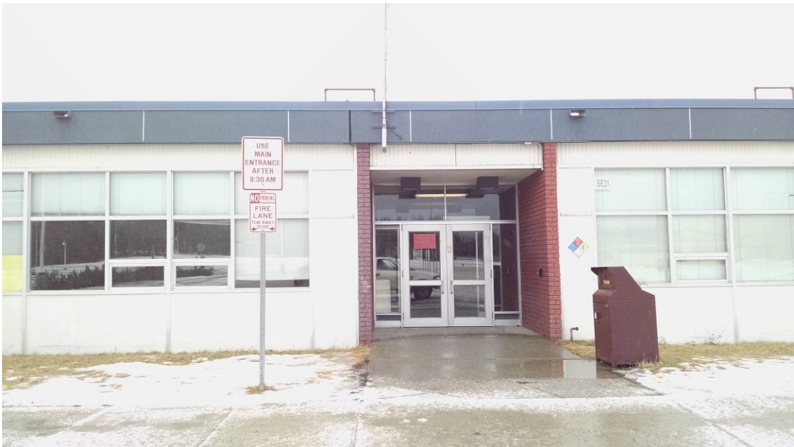
Figure 14: East High School main entrance (East)
