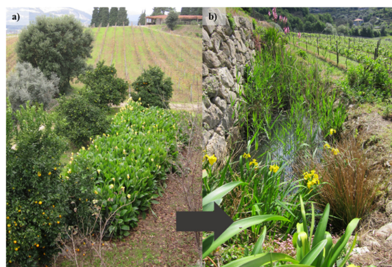
Figure 1. Constructed wetland (CW) (a) with a polyculture of ornamental plants for domestic wastewater treatment followed by a pond (b).
