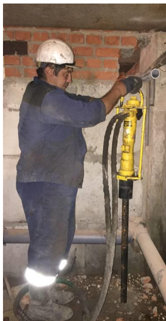
Fig. 4. Execution of jet grouting in the basement
