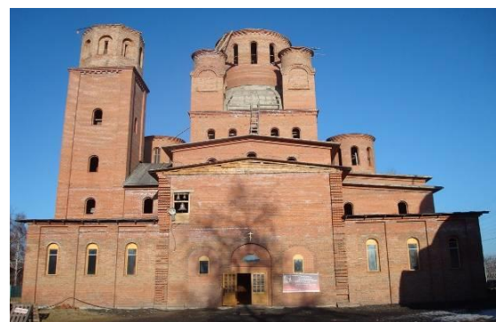
Fig. 1. View of church
