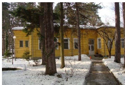
Fig. 3. View of pneumology 1 hospital building
