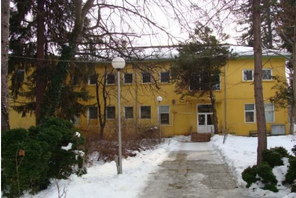
Fig. 4. View of pneumology 2 hospital building
