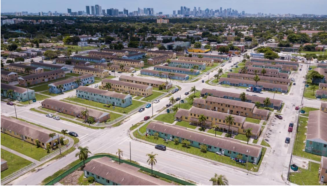
Figure 23. Public housing development in Liberty Square - Miami, Florida (Rodriguez & Hanks, 2019).
