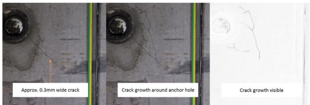
Figure 6: Detection and evolution of a crack between sample pictures (Stent et al., 2015).
