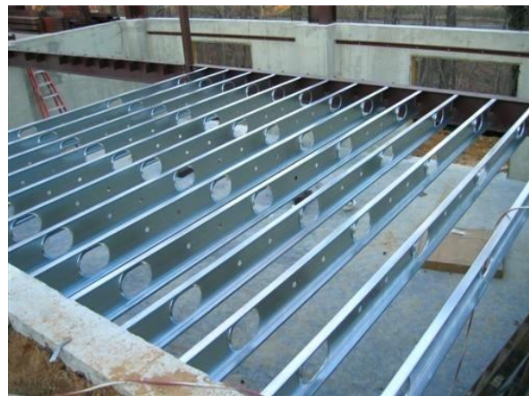
Fig 1.2: Cold-formed floor system (image courtesy of IMGLABS.co)
