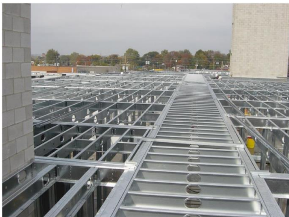
Fig 1.1: Cold-formed framing system (image courtesy of ClarkDietrich Building Systems)
