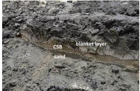
Figure 10 Irregularly eroded CSB with subsided blanket layer after failing in Test 2 (view in upstream direction). Length of the excavated CSB is approximately 2.5 m.
