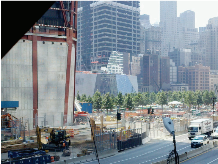
Figure 4.17. View of the reinforced concrete base of 1 World Trade Center with the deconstructivist façade of the 9/11 Museum in the background. Photo by Karla Kelsey, August, 2011.
