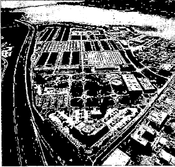
Figure 12a. Blue Plains Wastewater Treatment Facility.
