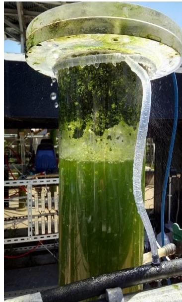
Fig. 46 Active water spray cooling system.
