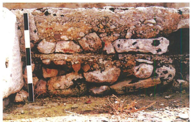
Figure 3. Successive bedding layers for floors inside room A (possibly the atrium) (photograph by Antonio Caselli).
