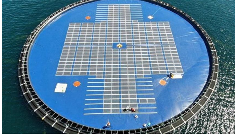
Figure 27. Swimming Solar Park by Statkraft, Albania
