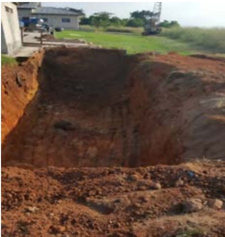
Figure 15: Clockwise from left, digging of soak away pit, filling soak-away pit with boulders, pit covered with sand, soak away pit covered with a polythene sheet (Photo: ILRI/Iheanacho Okike)
