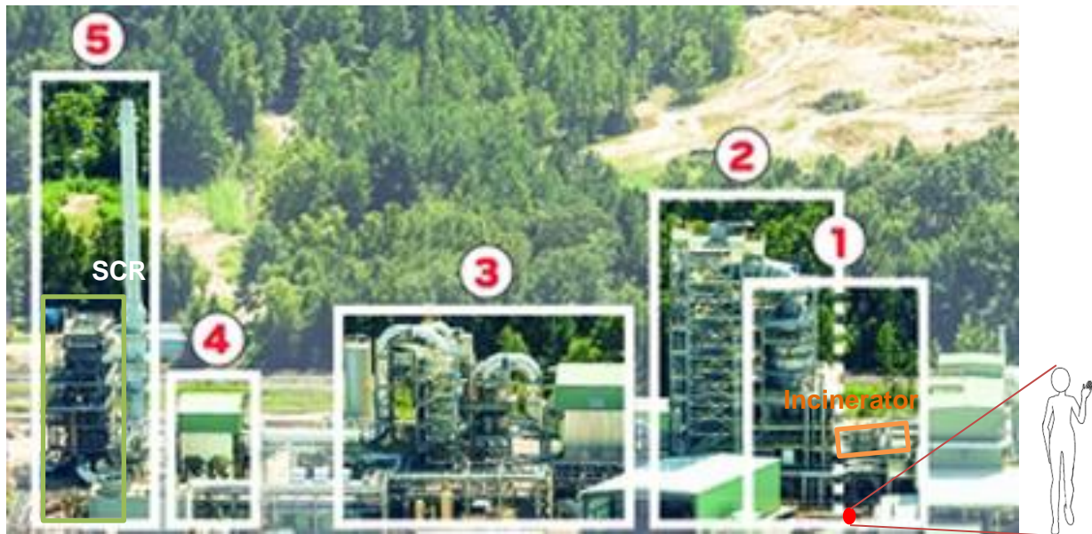
Figure 1-13. Clean Harbor Waste Incinerator. Adapted from [58].
