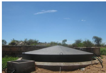
Figure 3. Typical example of a biogas supplied via flexible pipeline in India [48] (reproduced with permission from Reddy, 2015).
