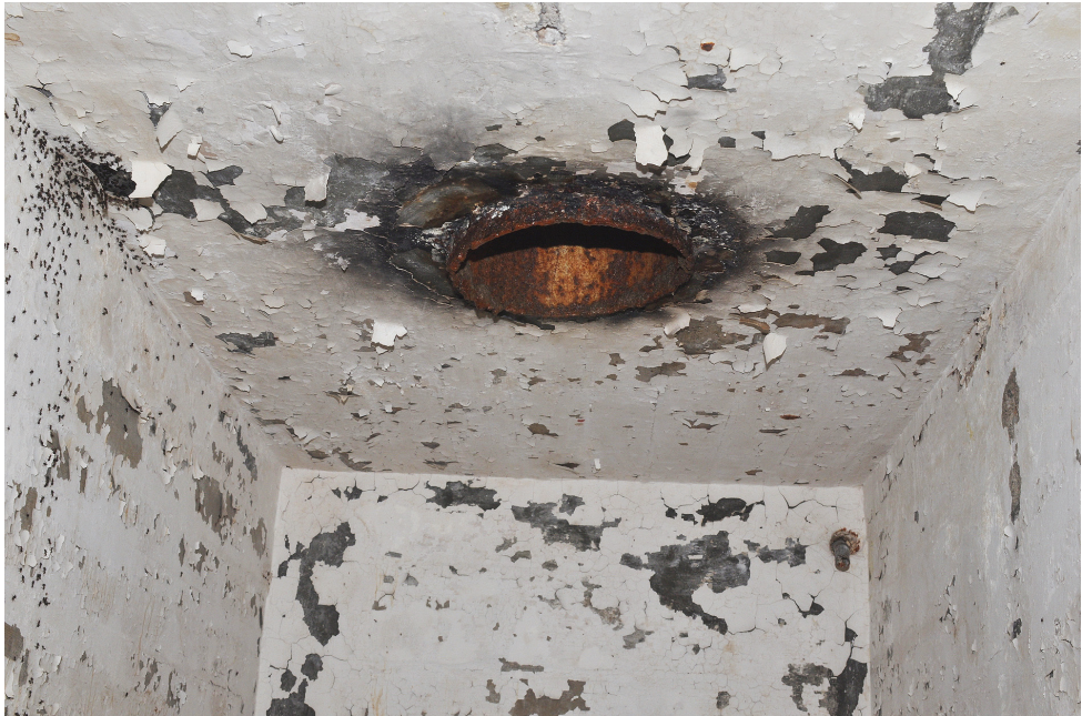
Figure 2. The upper part of the ant trail in Fig.1; the ants (on the left) were unable to move along the ceiling and thus could not reach the outlet of the ventilation pipe. Photo taken on 18.09.2016 (Wojciech Stephan).
