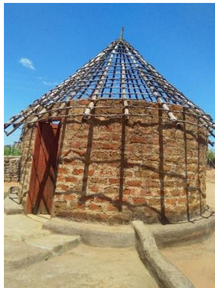
Figure 5.14: Support structure for a roof seen from outside
