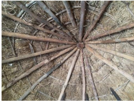
Figure 5.15: Inside view of thatched roof
