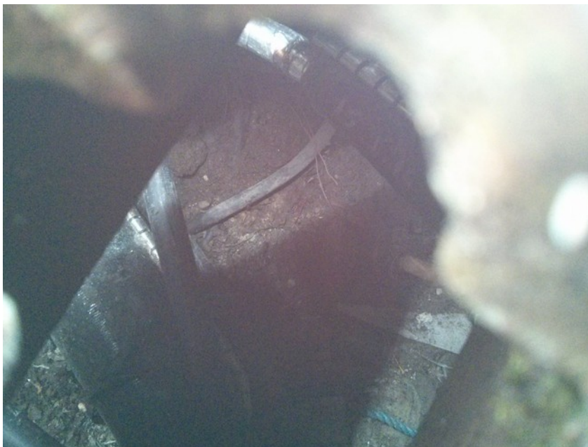
Fig.131 New Cloud Atlas, p.309 participants mapping network infrastructure. Photo: Laura Conerney; View of fibreoptic cables under Liverpool.
