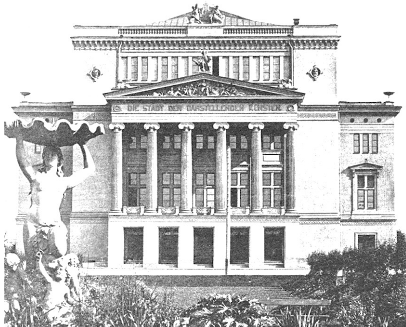
Figure 43. The First (German) City Theater, early 20th century – later the Latvian National Opera; note the text in German above the portico.
