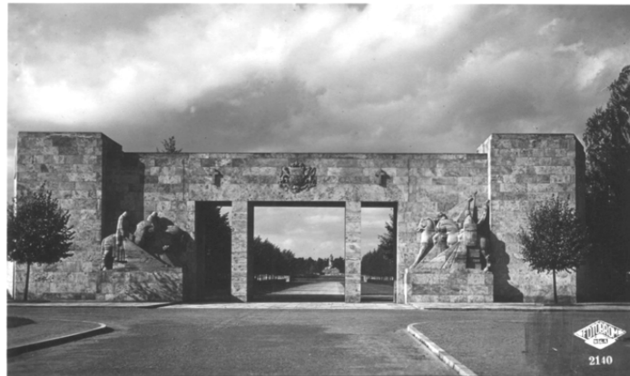
Figure 20. Gates to the Cemetery of the Brethren, 1930s.
