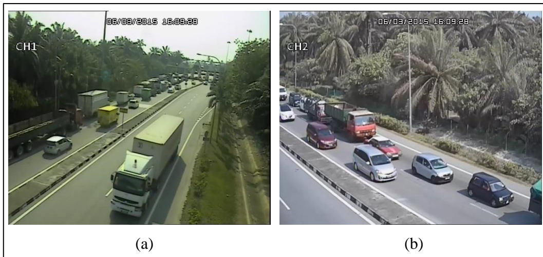
Figure 4.33 Screen capture for the maximum queue length condition when exceeding the camera view range at the exit of Jawi toll plaza; (a) Video recording of camera toward toll plaza, (b) Video recording of camera toward upstream lanes.
